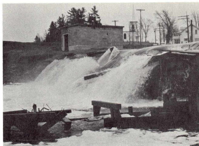
Bartholomew River dam, Blackville, New Brunswick, during spring freshet conditions.
