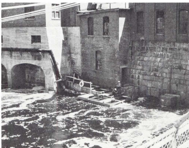
Fishway entrance (centre) at Milltown Dam on the St. Croix River, New Brunswick.
