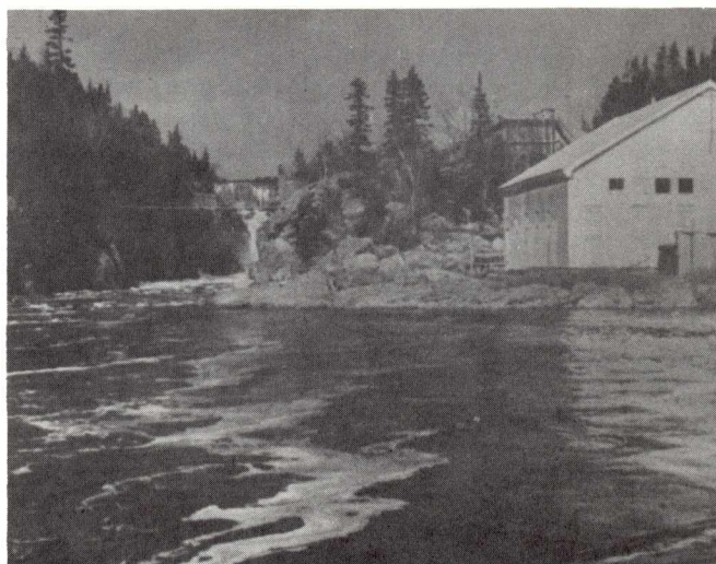
Liscomb Falls hydroelectric station, where fish passage facilities are to be constructed in 1976.
