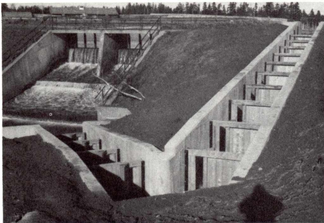
Newly constructed vertical-slot fishway at Scales Pond, Dunk River, Prince Edward Island.
