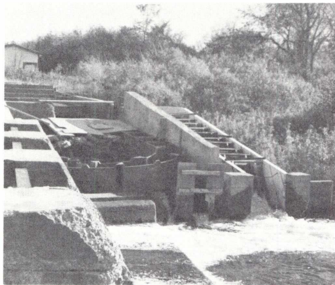
Spiral fishway (in new location) and Denil fishway on River Philip at Oxford Junction.
