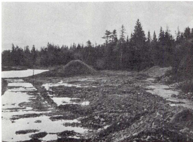
Gravel removal and channeling on River Tillard, Nova Scotia.
