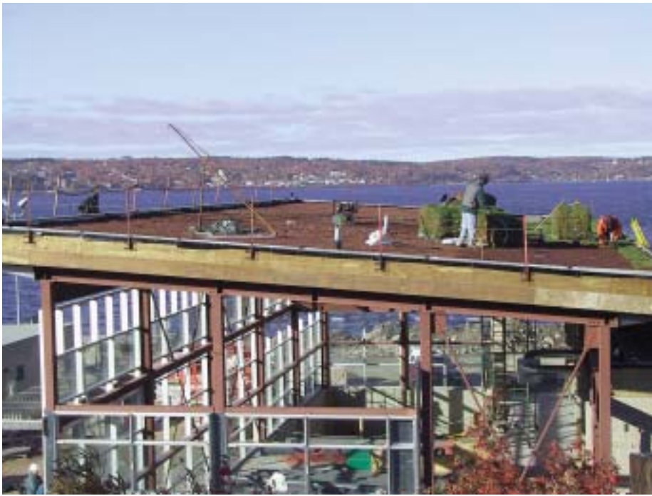
Installation of grass roofing material.
