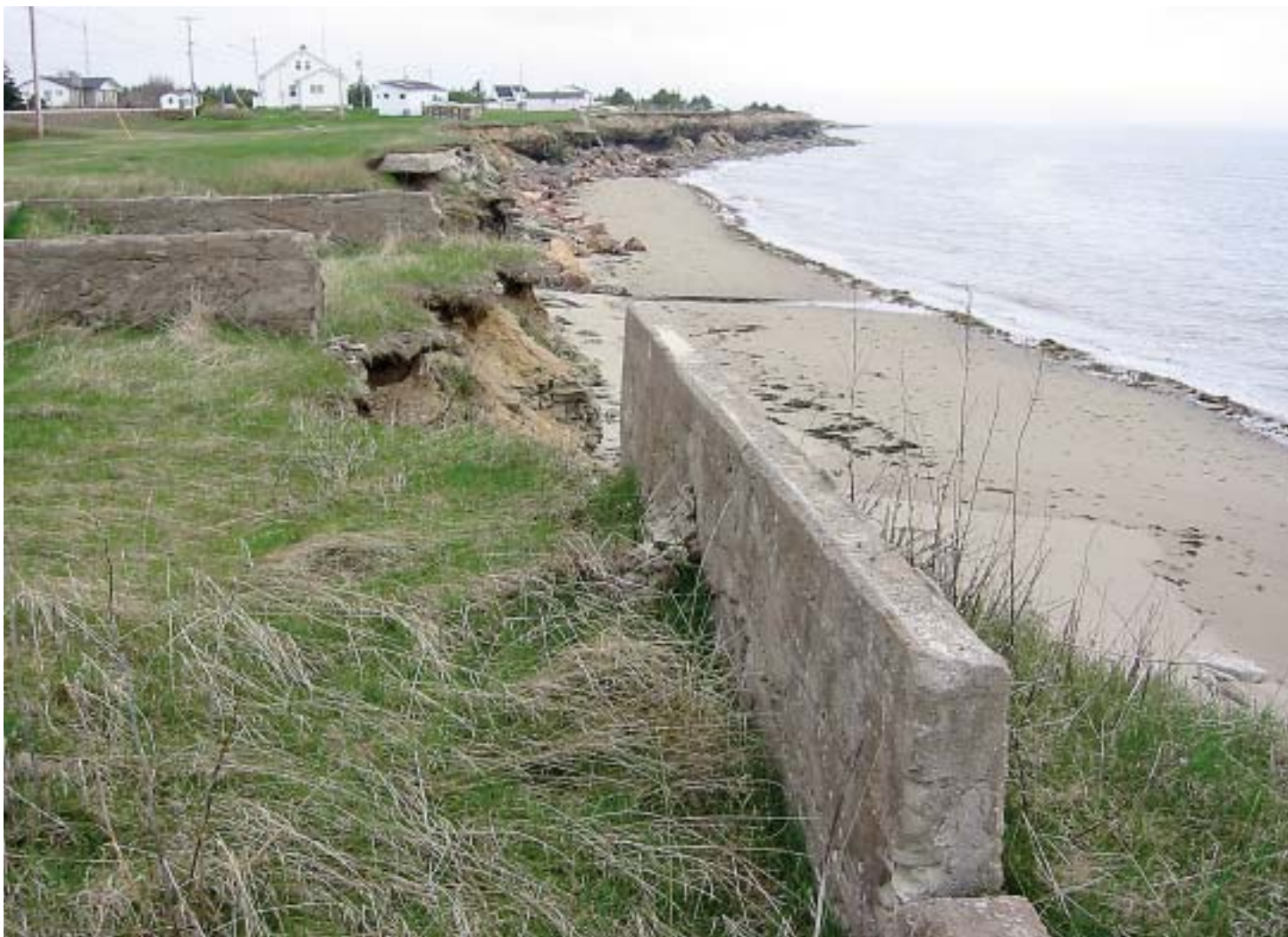
Abandoned and partly collapsed foundations attest to rapid erosion of low cliffs at Cap Lumière, NB. Other homes and businesses along this coast, including those in the background, are at risk from accelerated coastal erosion resulting from rising sea levels and other impacts of climate warming.
