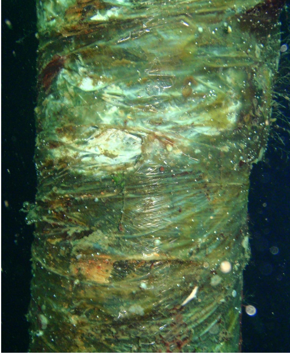
Figure 11. Encapsulation of a fixed wharf piling in Belleoram, Newfoundland, with sheets of plastic. Scale bar = ca. 2 cm. (Photograph credit: R. O'Donnell)
