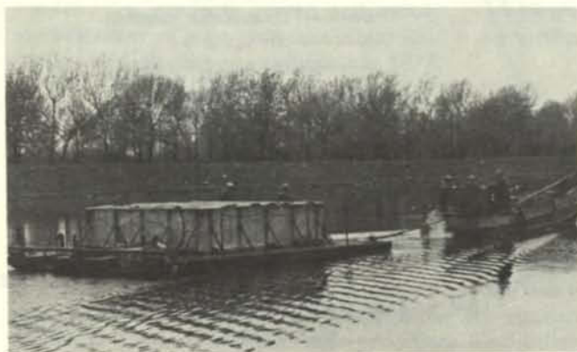
Figure 10. Alum application barge used on Fourth Welland Canal.
