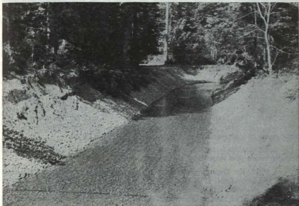
Spawning channel 2400 feet long and 20 feet wide, constructed adjacent to Big Qualicum River, B.C., in 1963.
