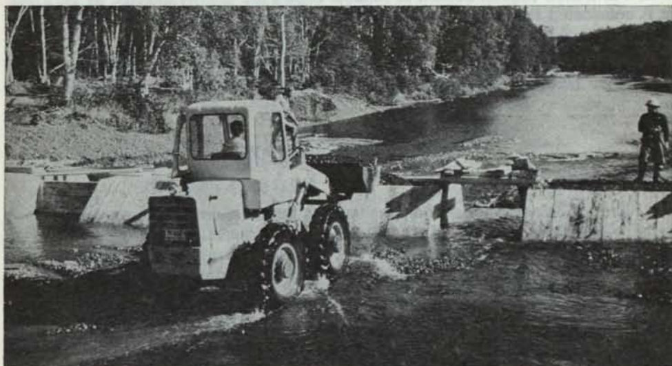
Weir construction, Indian River Spawning Channel, Newfoundland.
