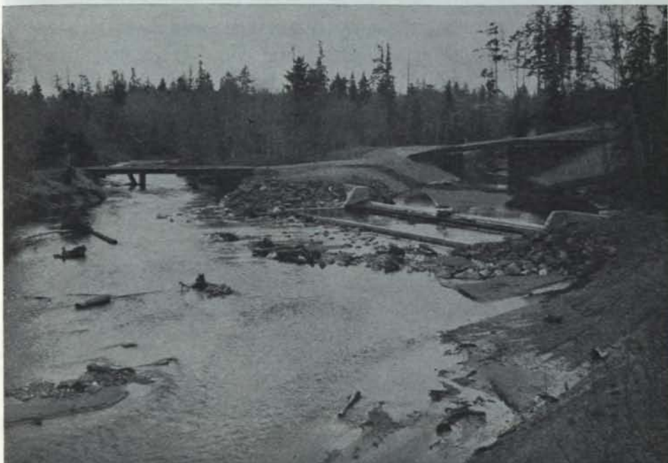
Confluence of Hunt's Creek flood channel with Big Qualicum River near tidewater. Note barrier structure in flood channel (right) to prevent salmon migration above this point, also bridge behind drop structure.
