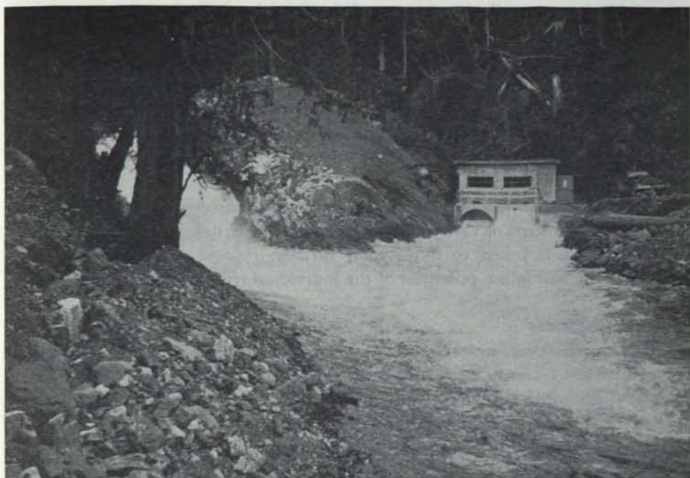
Valve house at foot of Second Falls for regulation of discharge. Big Qualicum project.
