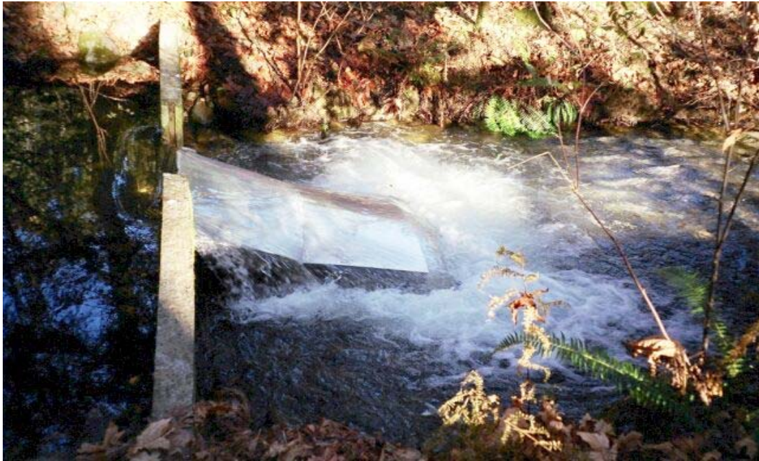
Photo 5. Chum salmon exclusion ramp installed in October 2003 at the lower end of the channel (0+317 m) which operates between October and December.
