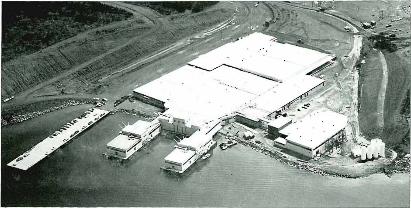
This aerial view of the new Lunenburg plant was taken before paving and roadways were completed.
