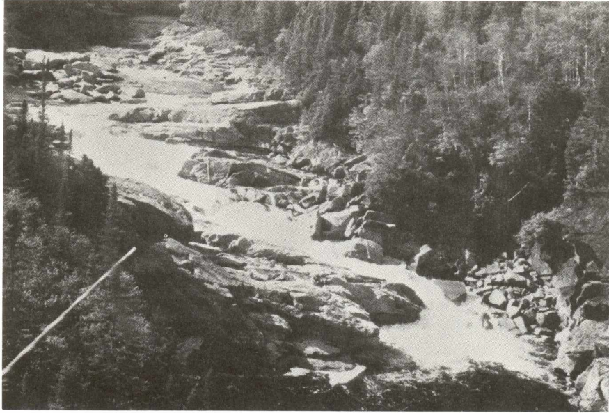
Fig. 26. White Bear river Construction site.
