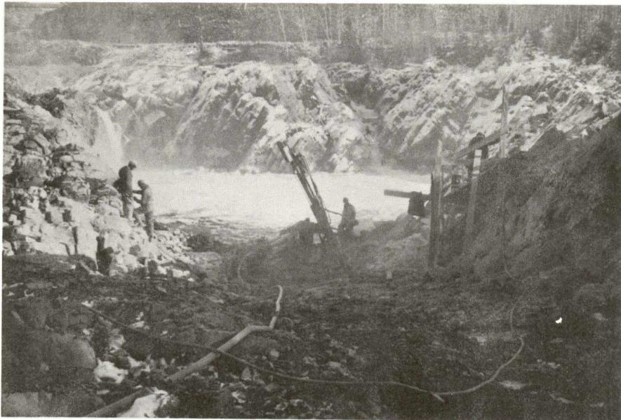
Fig. No. 25. Construction site, Grand Falls.
