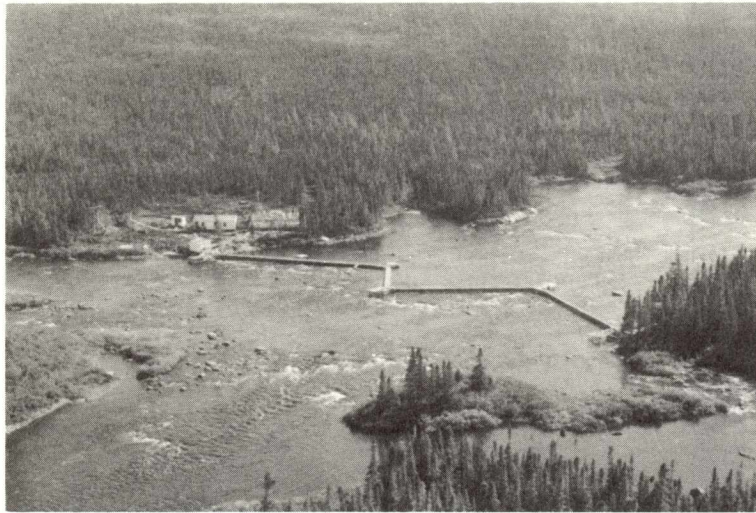
Fig. 11. General layout of Sand Hill River counting fence. The fence is approximately 500 feet long and the river is 410 feet wide. There are three adult traps and three smolt traps.
