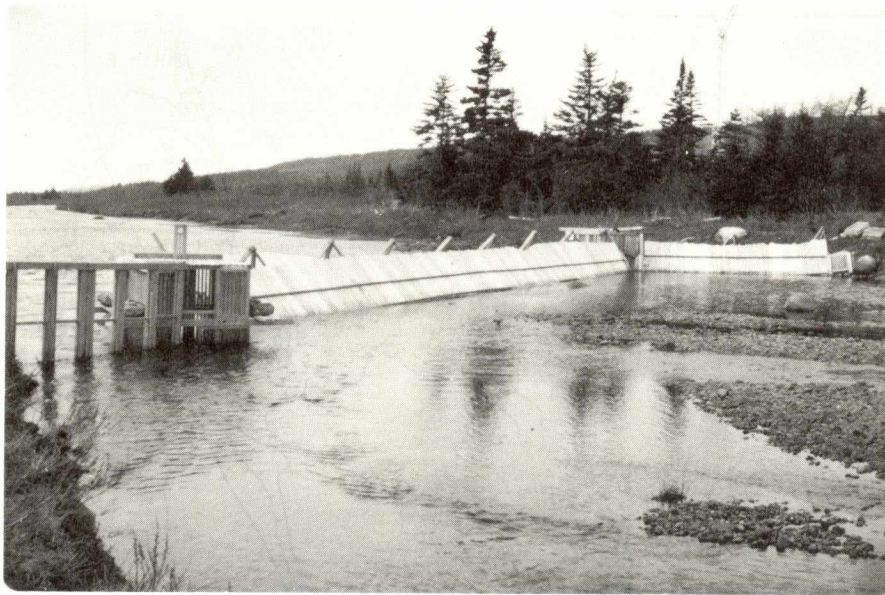
Figure 24. Conduit-type counting fence Come-by-Chance River, 1971.
