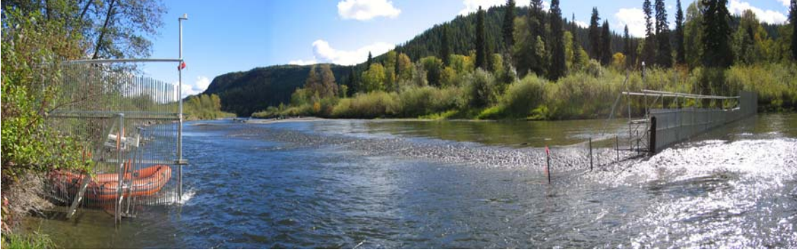
Photo 1. Cross-sectional view of the DIDSON hydroacoustic site on the Horsefly River. This downstream view shows the 7.4 m sectional fish deflection weir on the left-bank and a 37 m sectional weir on the right-bank. Active fish migration occurs in the faster flowing channel near the left-bank, between the two weirs. Photo taken by Juha Lilja on September 17, 2005.
