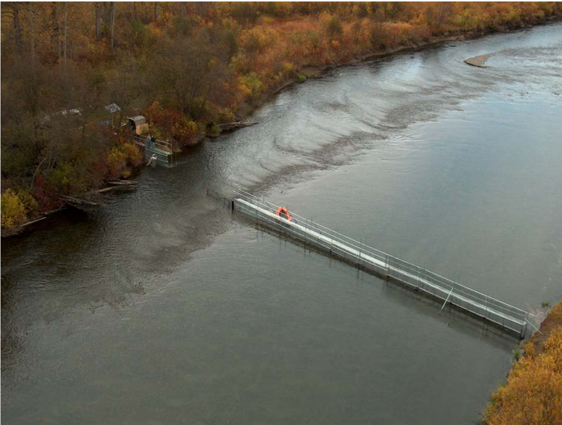
Photo 2. Aerial view of the hydroacoustic enumeration site on the Horsefly River. Note the extensive gravel bar running parallel to the left-bank creating a natural channel for fish passage between the two sectional fish deflection weirs. The river flow is from bottom left to top right in this photograph. Photo taken by Rob Dolighan on September 25, 2005.
