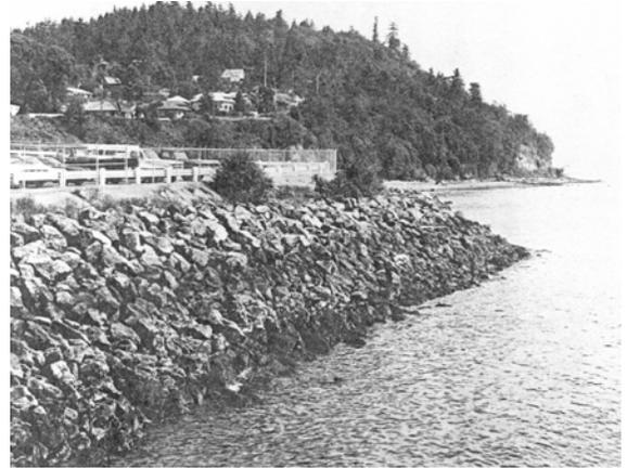
**Figure 5.12. Boulder revetment for landing**
