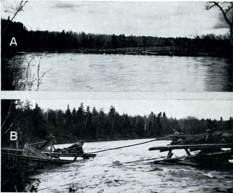
FIGURE 8. Pollett smolt counting weir after peak of a heavy spate (about 3000 cfs) in 1948. A —The weir extends downstream for 350 feet across 120 feet of stream width, starting at the large tree on the right; the tops of the 12-foot poles of the A-frames look like a farmer's fence against the right bank of the river. Notice saw-logs and other heavy debris piled against the fence up to the cat-walk which was 8 feet above the river bottom. B —Gap from which heavily ballasted and cabled trap box (8 feet wide \times 10 feet long \times 6 feet high) was carried away by flood.
