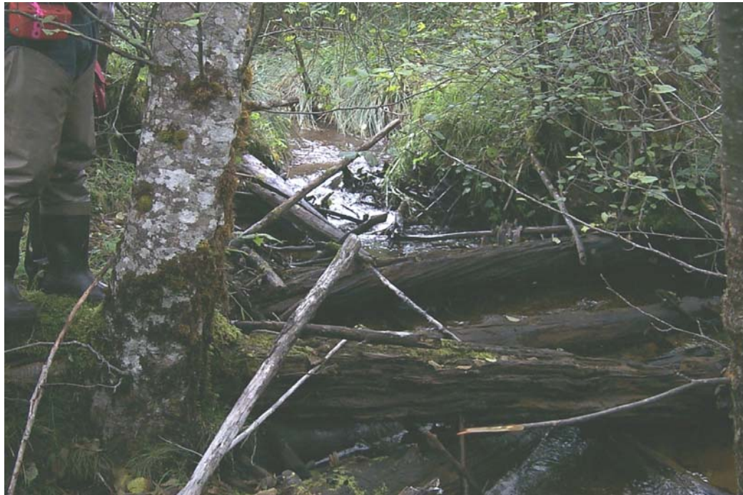
Photo 12: 0+200 m. Partial barrier to fish passage.
