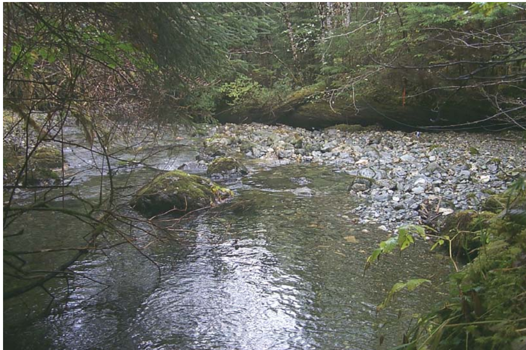
Photo 10: 1+350m – Looking UP from previous LWD jam at site for construction of rock line. This will divert water towards the side channel.
