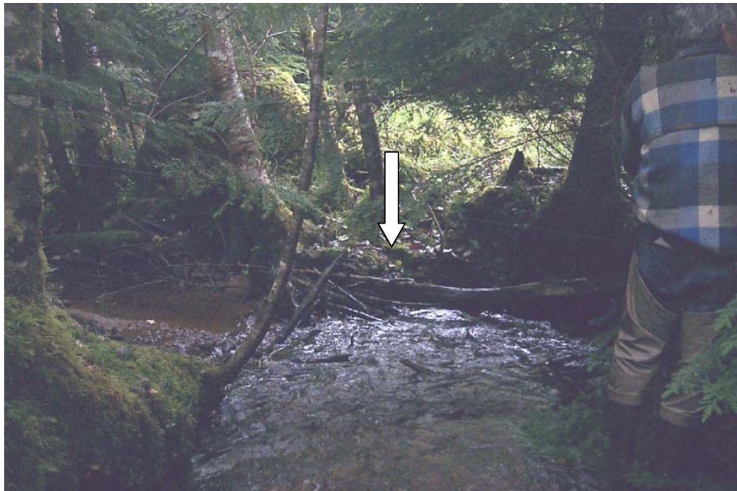
Photo 6: 0+100 m. Looking DN from mid-channel at SWD to be manipulated (arrow). Creek flowing under large stump seen to the left of the arrow. This results in blocked passage on the UP side.
