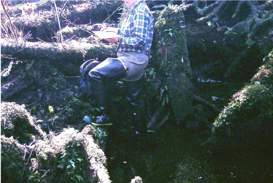
Photo 7: 0+067m. Looking upstream from the right bank at numerous suspended cross logs and SWD.
