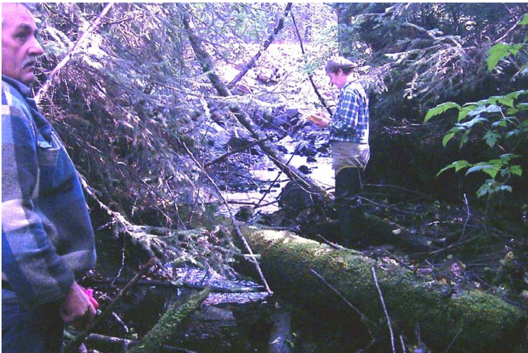
Photo 10:0+100m. Looking upstream from the left bank at SWD creating partial barrier to pinks.
