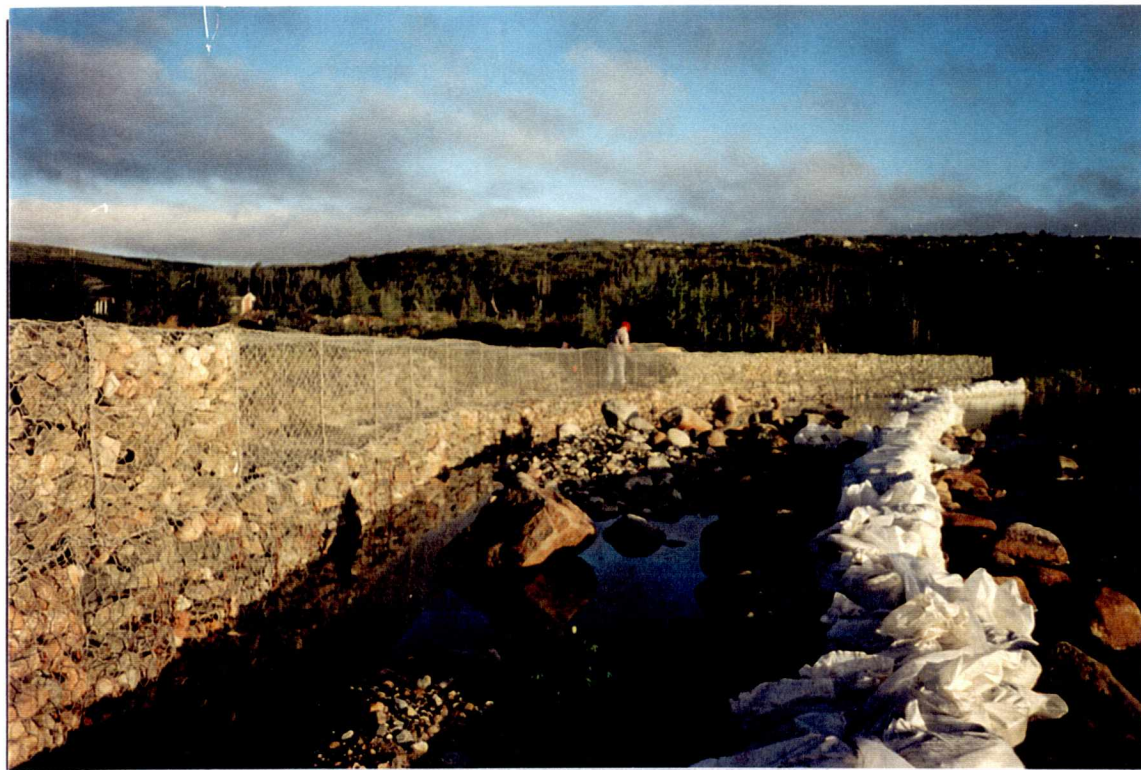
Stretching and placement of gabions on Top Pond Brook.
