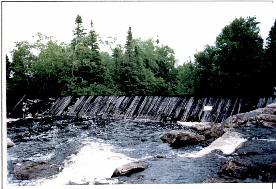
Old diversion dam before construction (downstream).
