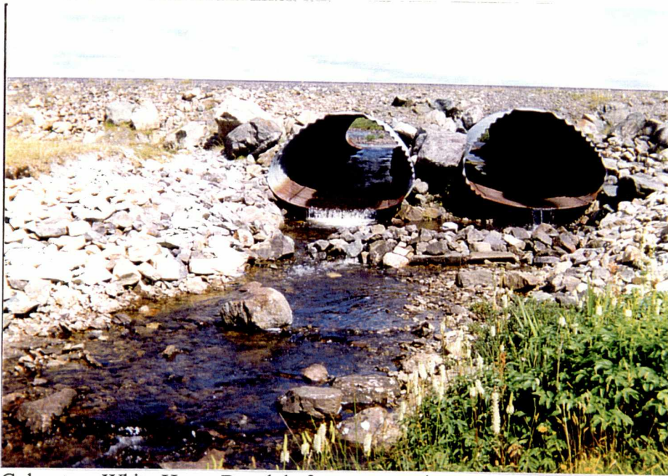
Culvert on White Horse Brook before stone weir was completed.
