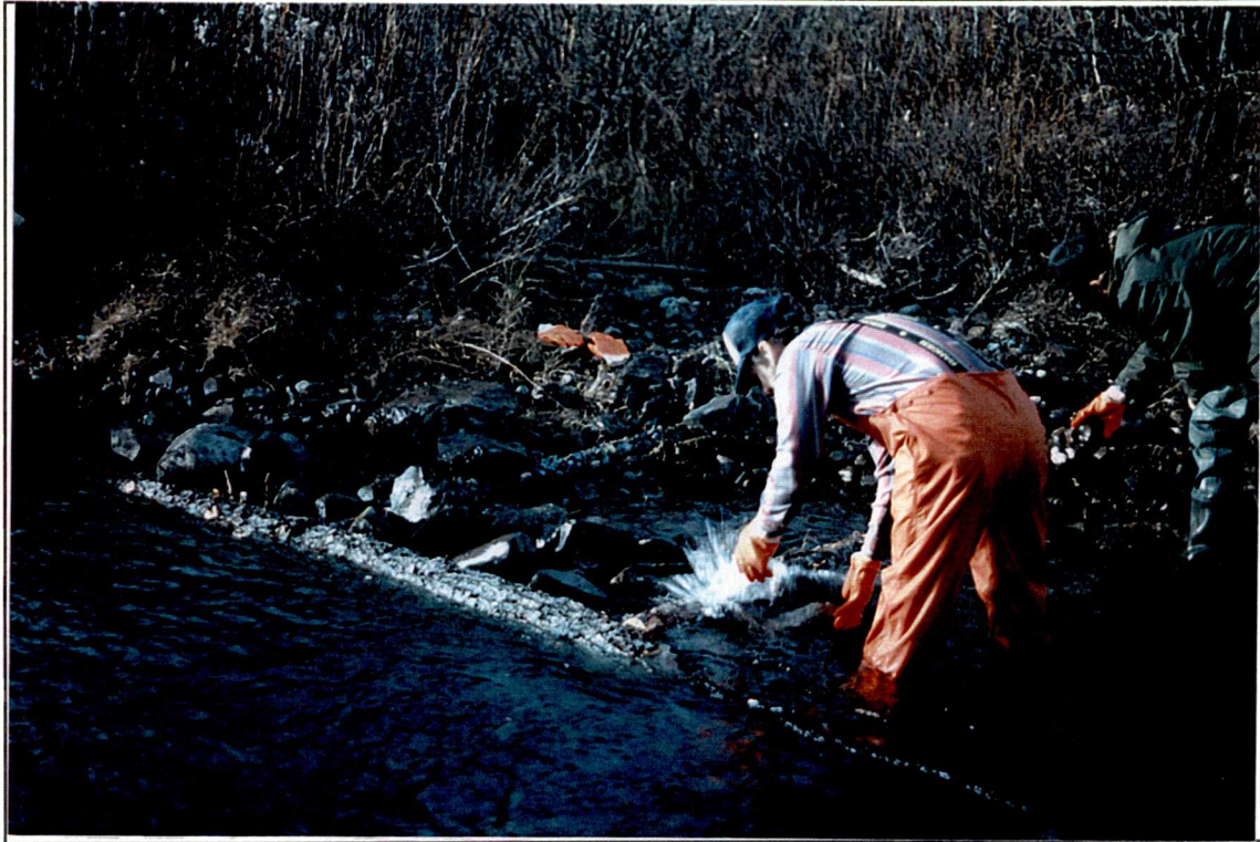
Installation of low head dams on Salmon River.
