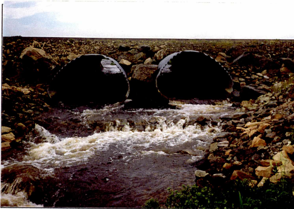
Culvert on White Horse Brook after stone weir placement.
