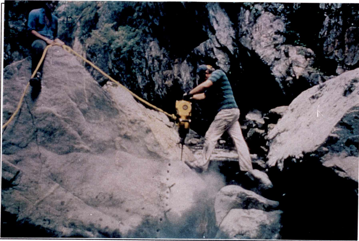
Drilling rock on Big Dead Wolf Brook prior to blasting.
