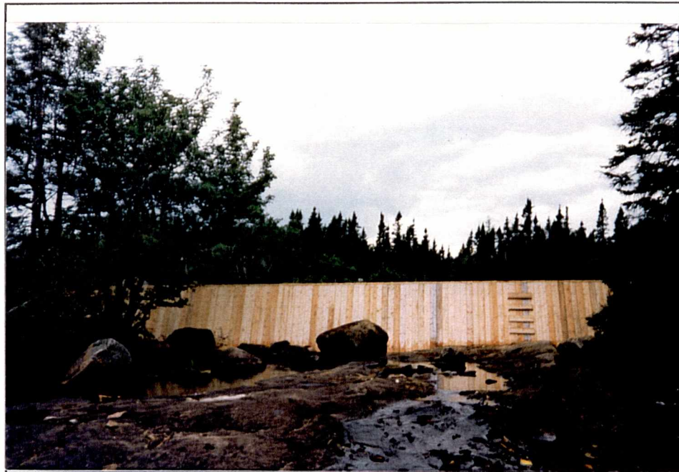
New Diversion dam (upstream).
