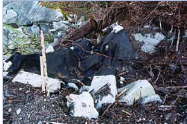
Photo 26. Poor runoff control through lack of maintenance of existing structure
