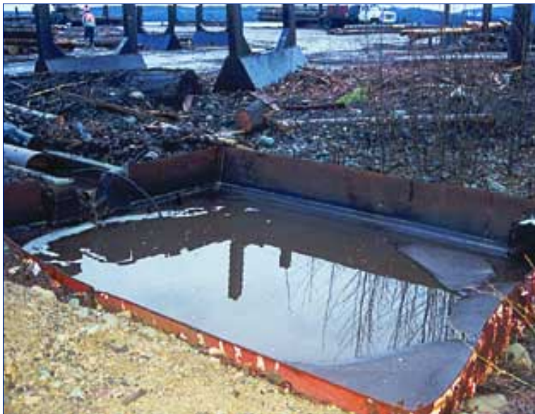
Photo 25. Runoff control (sediment settling pond)
