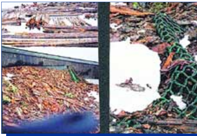
Photo 27. Debris net in position below a metal skid
