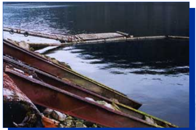
Photo 28. Containment booms in place at a skidway
