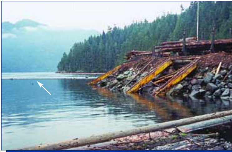
Photo 4. Log dump located on steeply sloped shoreline, with logs used for debris containment visible in the distance
