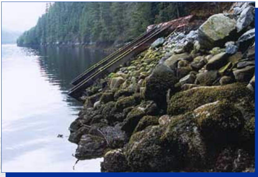
Photo 33. The colonized riprap fill along the shore should not be disturbed when the site is decommissioned
