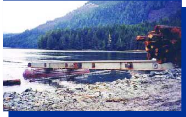
Photo 14. Log dumping using steel skids, skids span intertidal area
