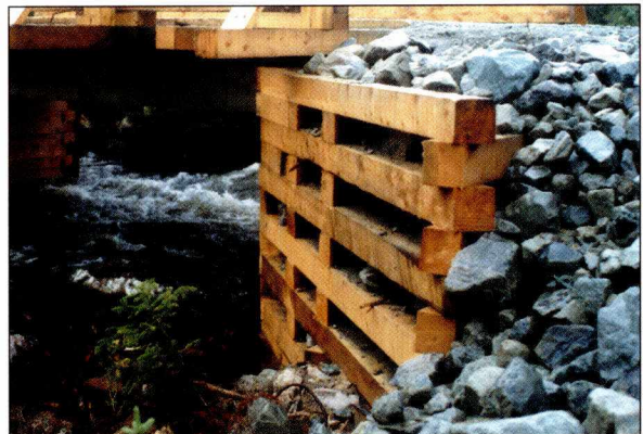
Infill materials for timber cribs.
