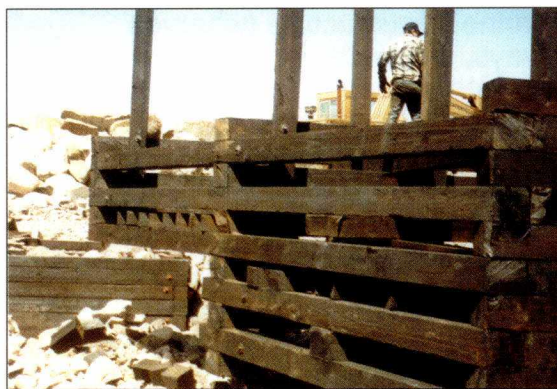
Timber crib construction for marine environment.
