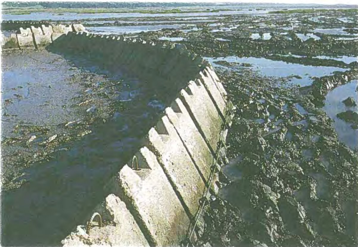
Sediment confinement structure, Rivière-du-Loup Bay.
