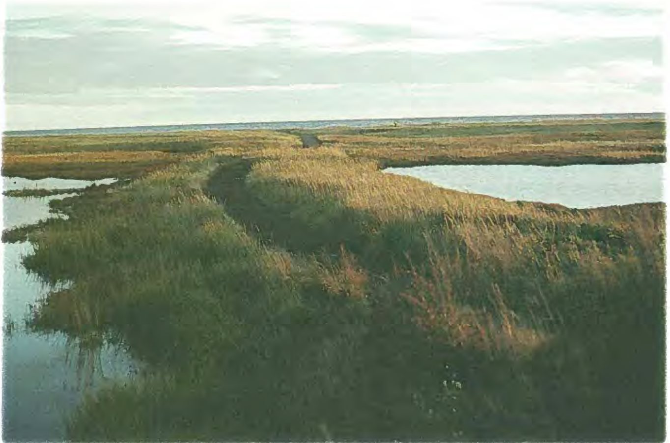
Caen Road, embankment of the New Carlisle barachois.
