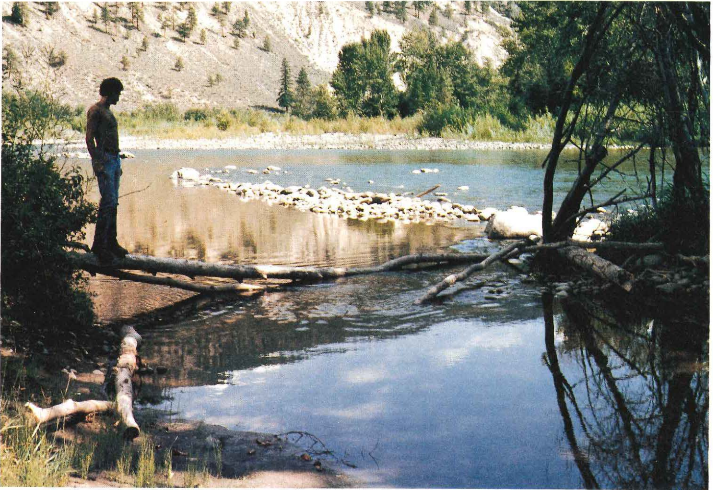
A wing diversion built of rocks channels a portion of the Nicola's flow directly onto alfalfa fields located "downstream."
