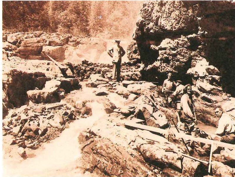
In May 1927, construction was started on a fishway past Stamp Falls.
