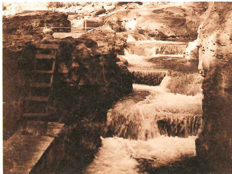
In September of the same year, the fishway was completed. Sockeye could now pass Stamp Falls more easily on their return to Great Central Lake. Photos: DFO Files
