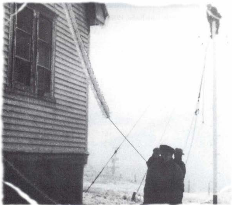
Camperdown staff repairing antennae after an ice storm, 1938. (W.H. Wooding)
