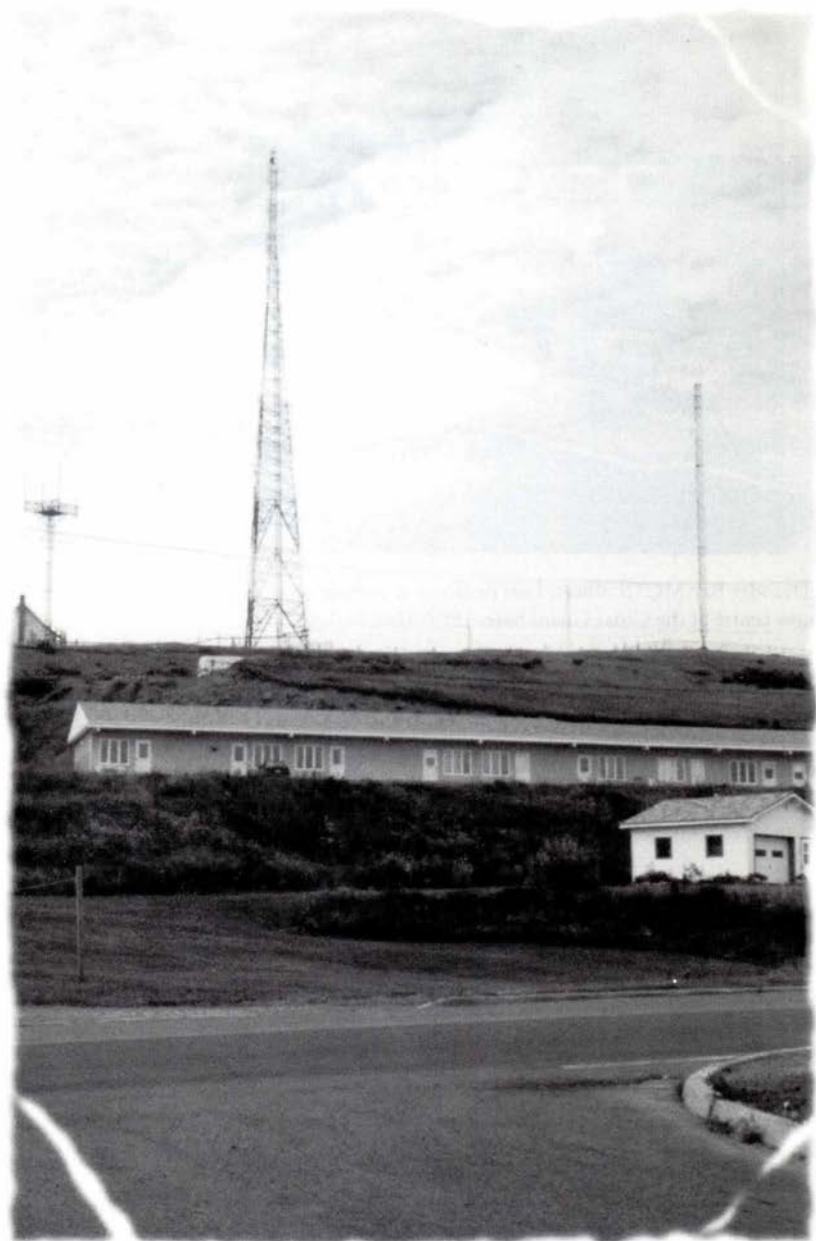
Cap-aux-Meules MCTS's transmitting and receiving antennae. Small house, top left, is the ex-Marconi wireless station, 1997. (Gisèle Bettez)
