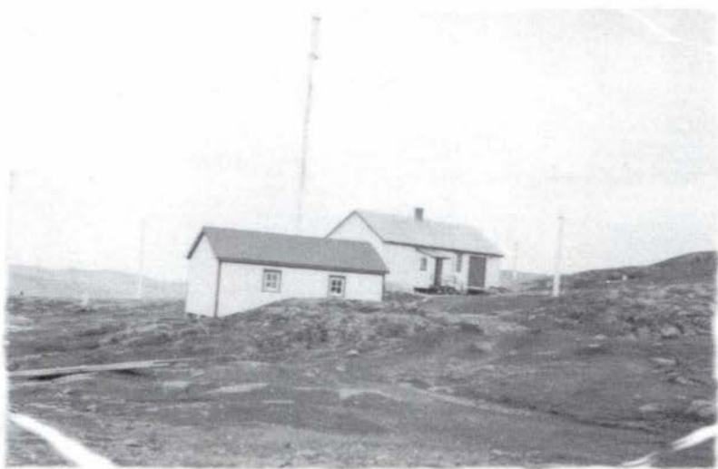
Outside view of Marconi station at Belle Isle. The longer building housed the radio station. The four short masts supported the direction-finding loops. The longer mast in the centre supported the main antenna, 1956. (Samuel Johnson)
