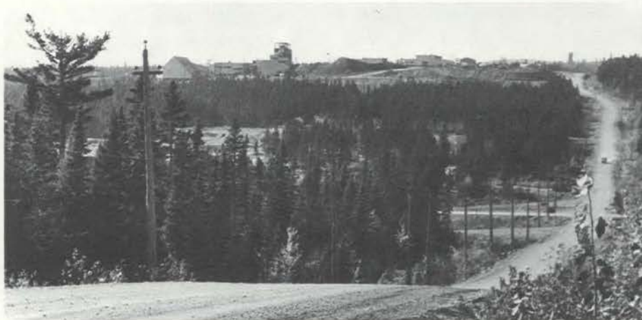
Mines, even when some distance removed from a stream, can contribute fish-killing poisons. Rain run-off from the scarified land and the roadbeds made of low grade ore waste from this copper-zinc mine can cause death of young salmon and turn back migrating adults in the main river more than 20 miles away.
