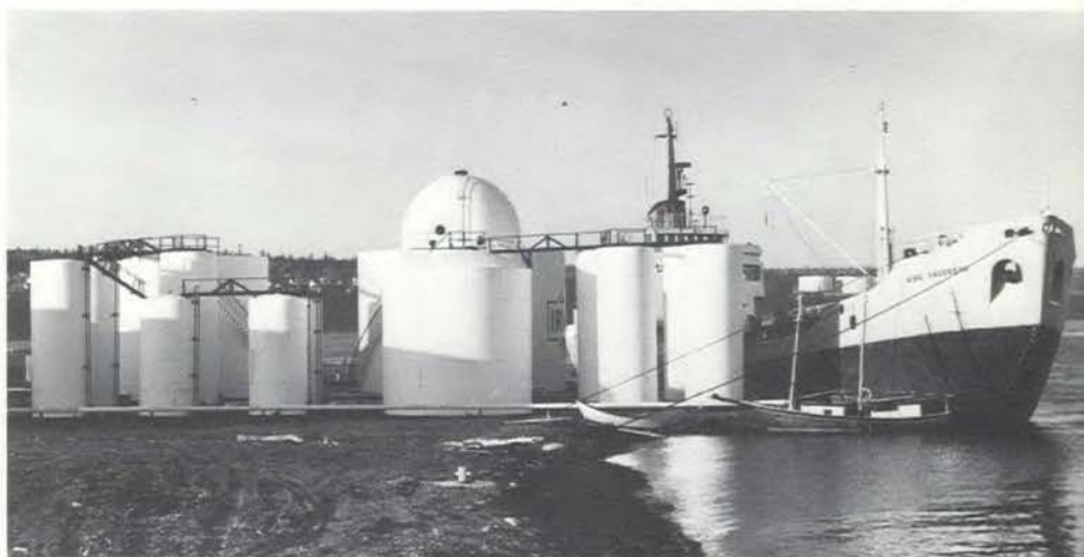
In some areas, oil storage depots such as this are placed on concrete sumps which prevent oil spillage from soaking into the ground and thence the water. The Miramichi estuary has several depots unprotected by oil-proof sumps and at least two large oil slicks occurred on the estuary this past summer when oil was being transferred from tankers.
