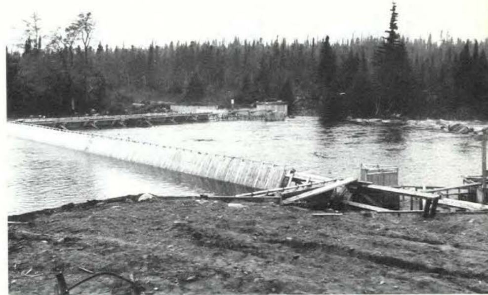
Overall view of the Salmon River counting fence showing two smolt traps downstream and one adult trap in the apex upstream.
