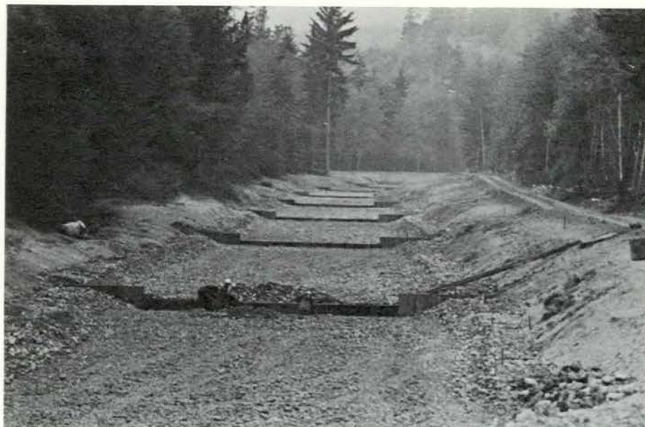
Photograph taken during construction of the spawning channel shows dividers between the sections.
