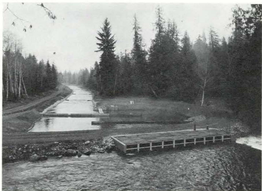
Completed spawning channel, showing intake and settling pond.
