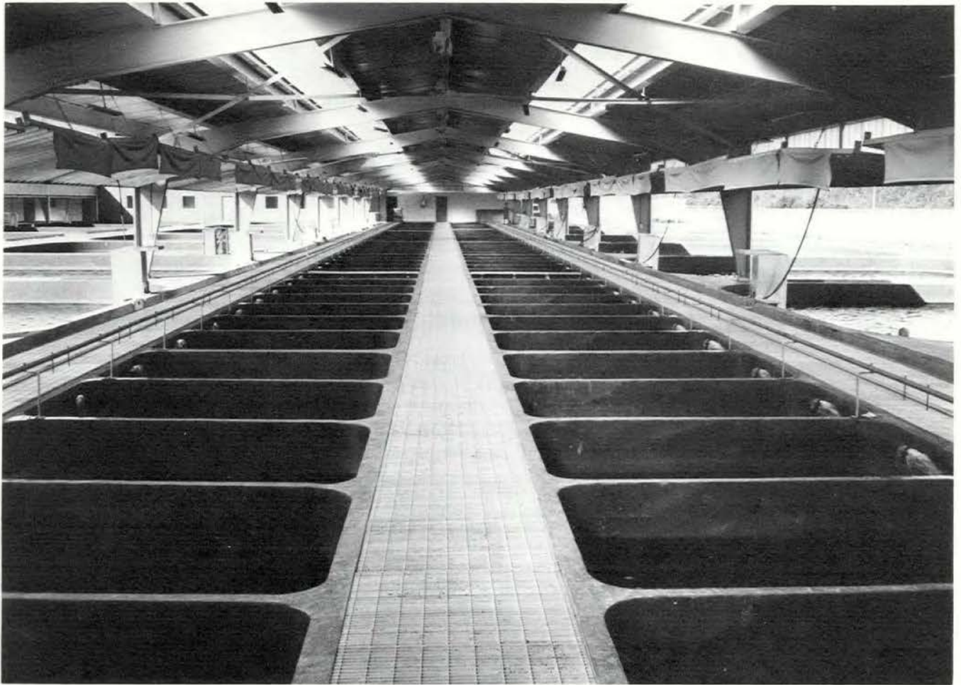
A section of the rearing tanks at the new Mactaquac fish hatchery built by the New Brunswick Power Commission and operated by the federal Department of Fisheries.
