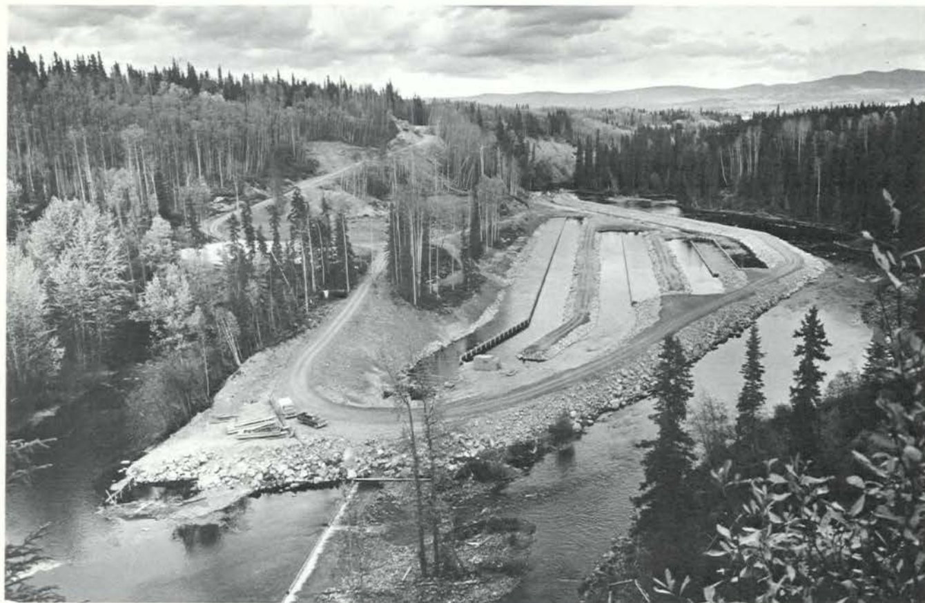
Panoramic view of the sockeye salmon spawning channel adjacent to the Fulton River, completed in 1965.
