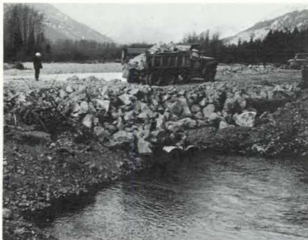
Dumping rip rap around the culverts installed between the Squamish River and Judd slough.
