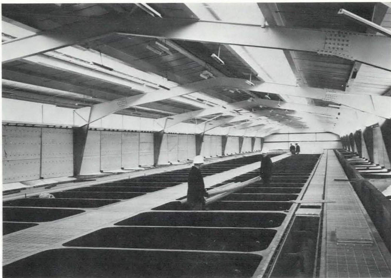
Salmon rearing ponds in one of the buildings in the almost-completed Mactaquac station.
