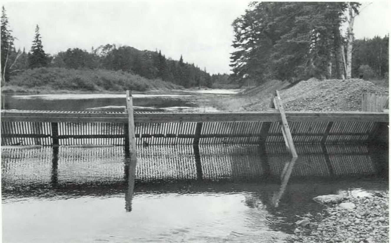
Diversion fence directs Indian River salmon toward controlled flow spawning channel beyond right bank.
