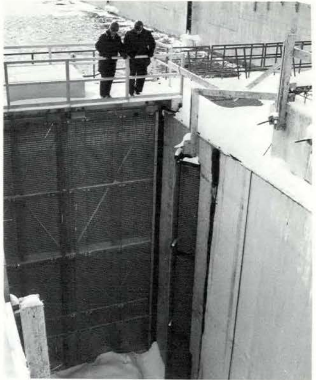
Close-up view of the salmon trapping facilities at Mactaquac hydro-electric dam.
