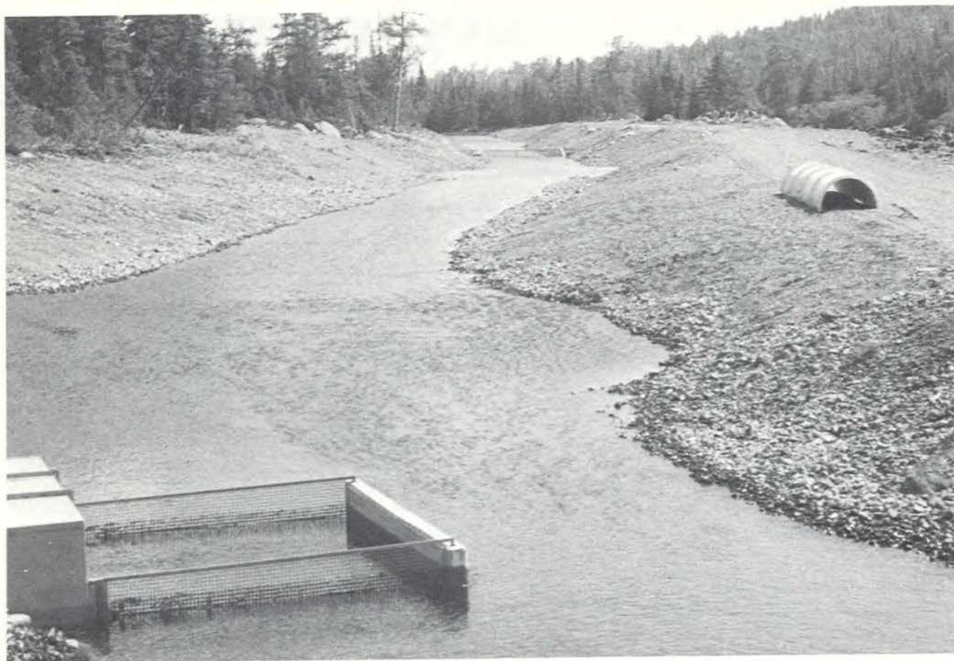
A down-river view of the newly-excavated Noel Paul Brook spawning channel, showing observation chamber (left foreground) designed to observe spawning habits of Atlantic salmon.
