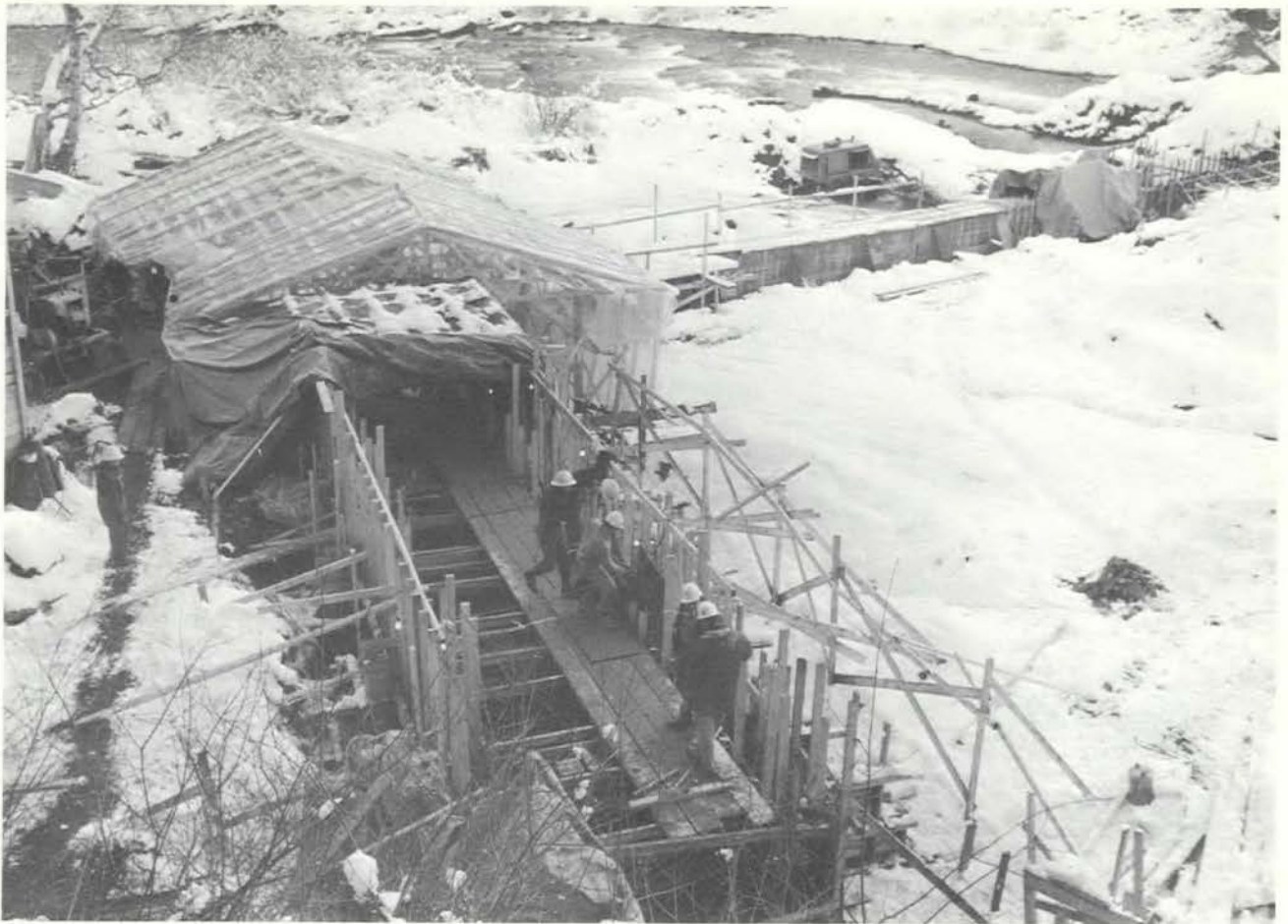
Meziadin fishway and barrier dam under construction, December, 1965.
