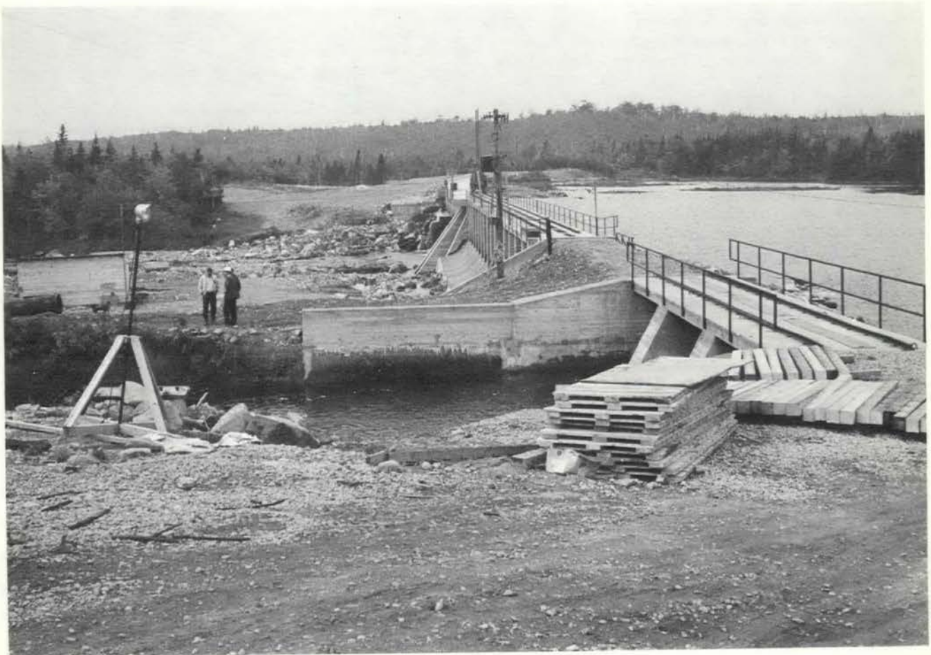
Construction of power dams such as this on East River, Sheet Harbour, N.S., dealt a death blow to Atlantic salmon in the river. A long-term rehabilitation project by the federal Department of Fisheries is aimed at restoring salmon to the river.
