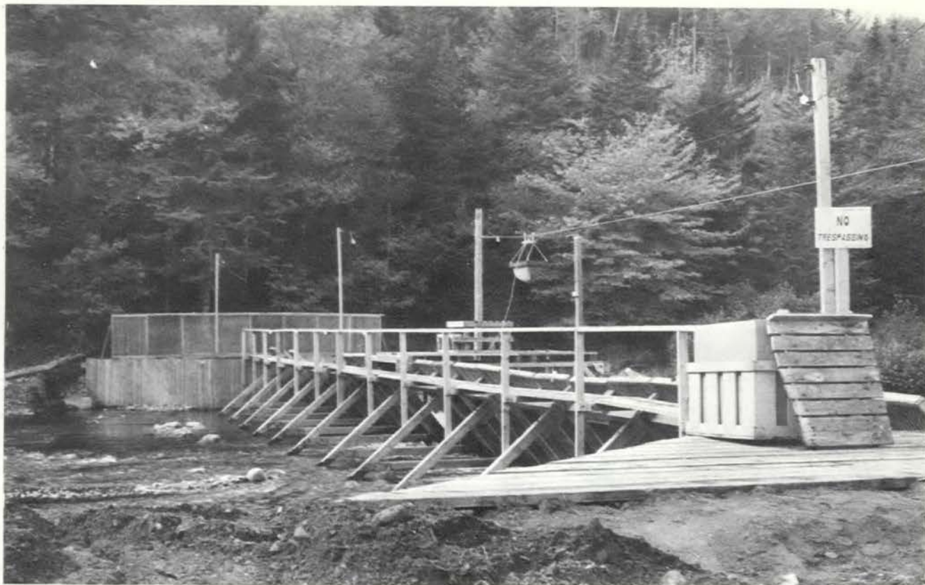
Fish counting and guiding fence on West River, N.S.
