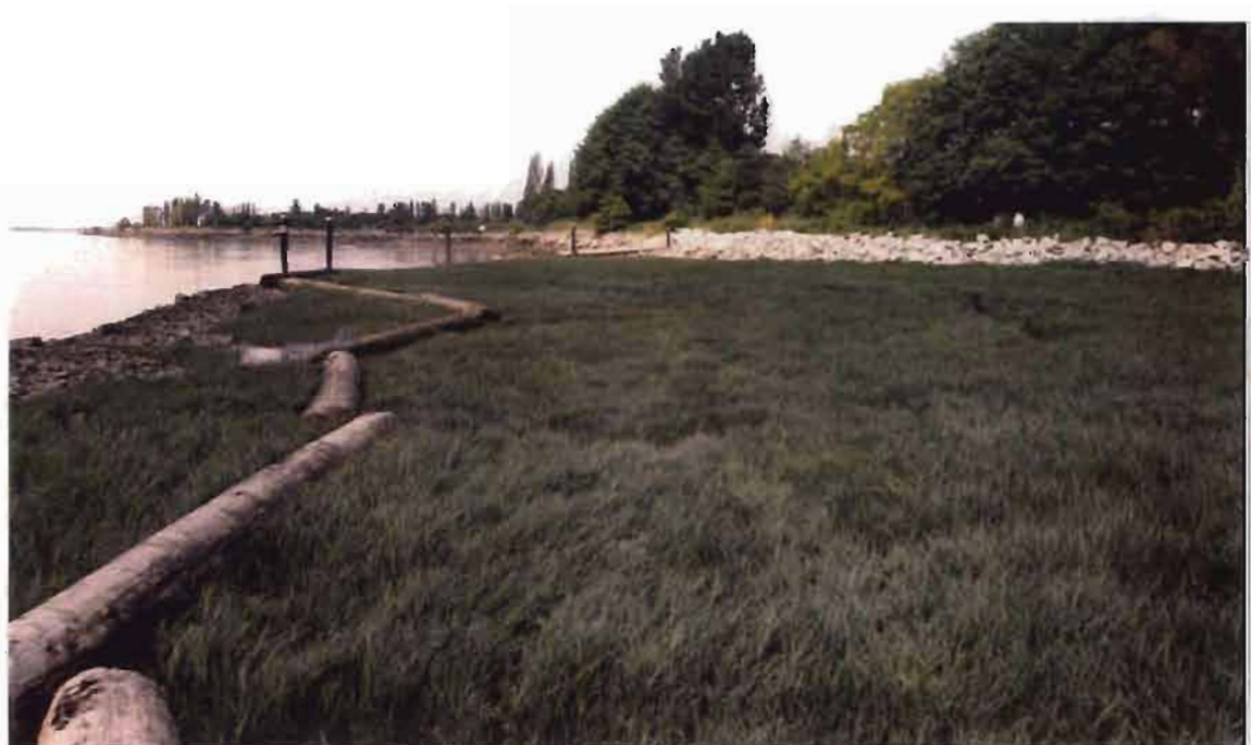
Figure 8. DI1 compensation site in the North Arm (see Figure 2). Protective log boom prevents debris (e.g., driftwood) from destroying vegetation. Photographed 96-06-03.
