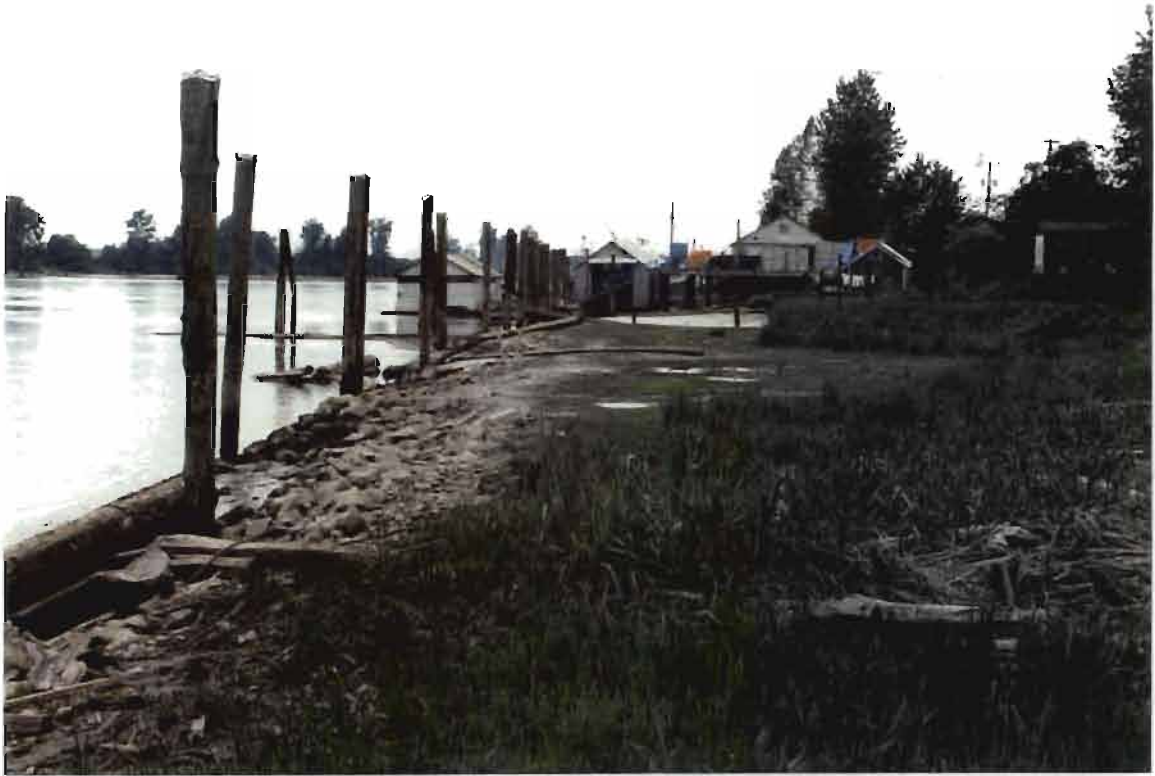
Figure 9. AC4 compensation site in Annacis Channel of the South Arm (see Figure 3). Marsh planted in 1991. However, excessive debris in the marsh area demonstrates a failed log boom. Photographed 96-06-03.
