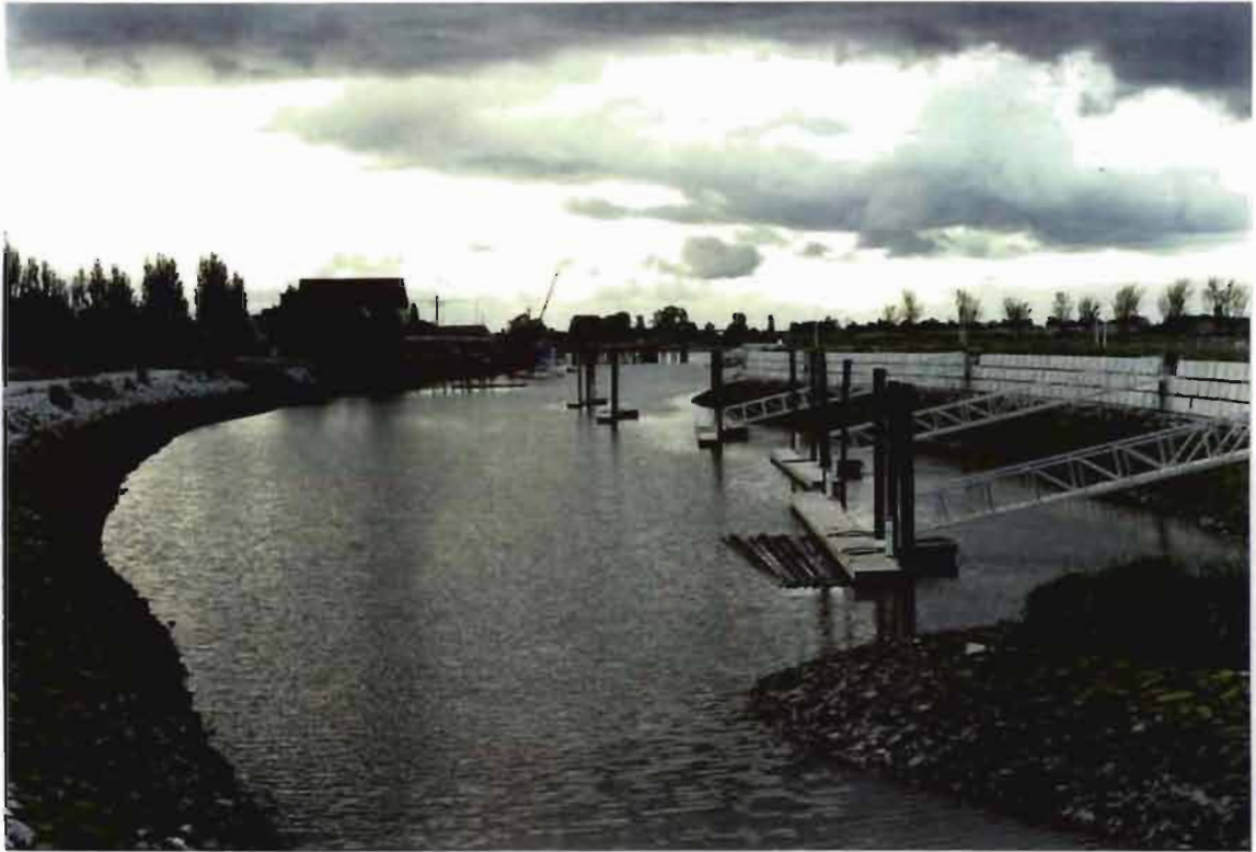
Figure 11. DI3 disrupted site at Deering Island in the North Arm (see Figure 2). Habitat loss due to placement of riprap revetment used to stabilize shores where residential development has occurred. Photographed 91-06-12.
