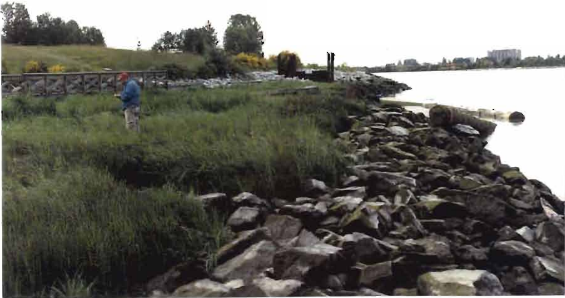
Figure 5. ANI compensation site located in the North Arm (see Figure 2). Riprap placed along perimeter to prevent erosion of marsh and vegetation planted in 1986. Photographed 91-06-12.
