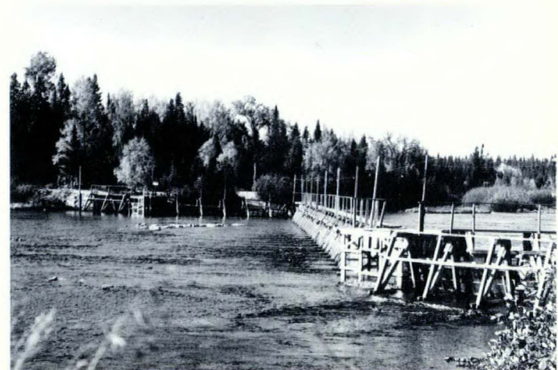
Important in management of fish resources, fish counting fences provide data used to estimate population sizes. This fence has been used for counting migrant salmon on the Northwest Miramichi River since 1950.
