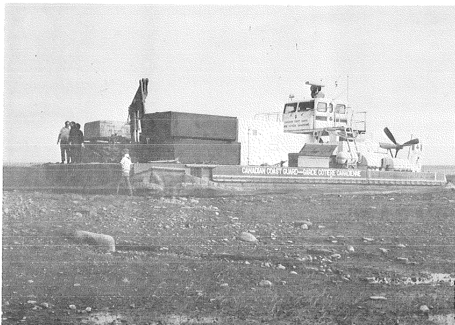
Delivering Building Supplies, Diesel Generator and Fuel Tanks for Construction on Ile Richelieu Light Tower Figure 9
