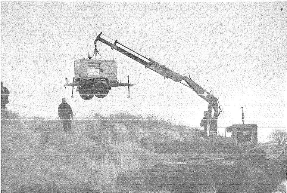
Figure 8 - Transporting Diesel Generator to VTM Station at Ile Grossbois
