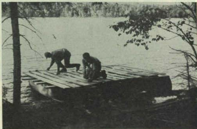
Building raft on two canoes at Camp Lake.
