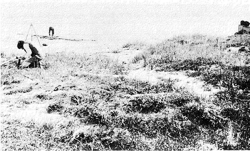
Setting a bench mark, and burying capillary tubing for pressure tide gauge at Liverpool Bay, N.W.T.
