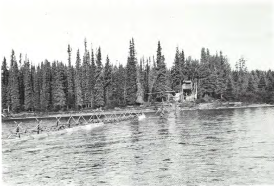
Plate 19. Counting fence on the Nisutlin River (river 400 ft. wide at this point with a discharge of 3000 c.f.s.)
