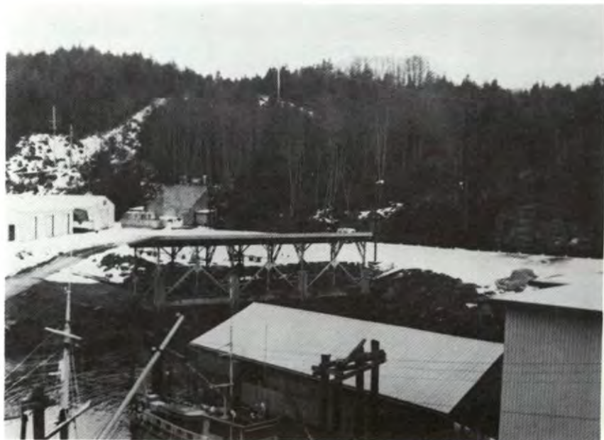
Plate 25. Prince Rupert Marine Station after levelling.
