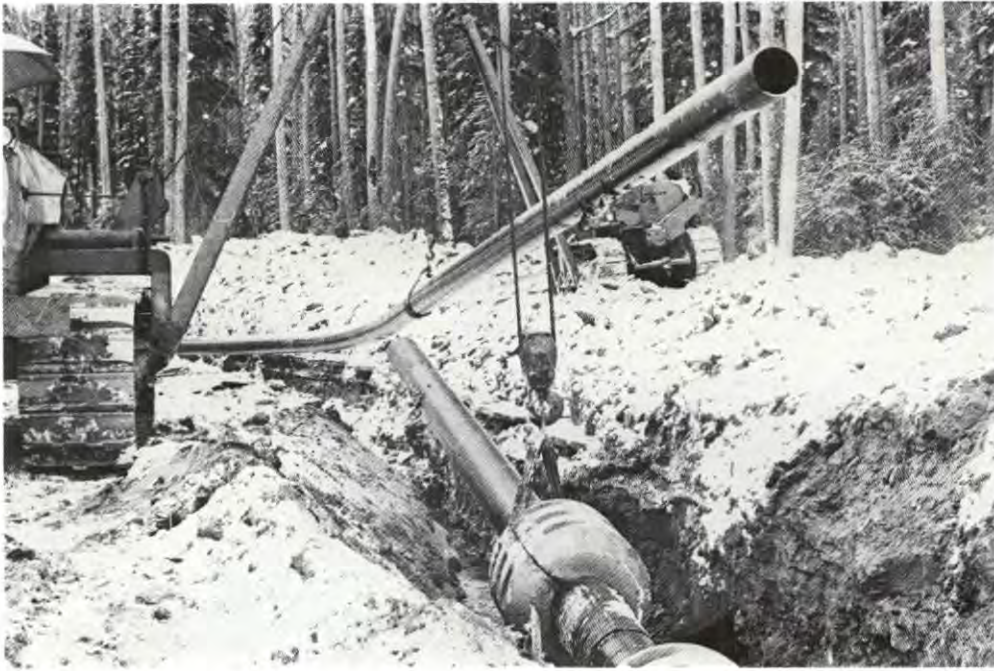
Plate 14. Beaver River - Pointed Mountain Pipeline.
