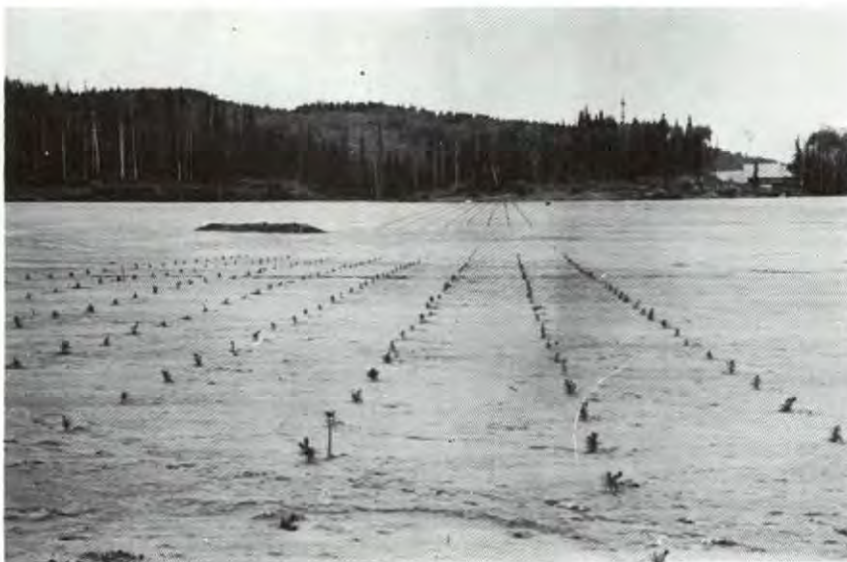
Plate 34. Granisle Copper tailings pond no. 1 - reclamation with evergreen trees.
