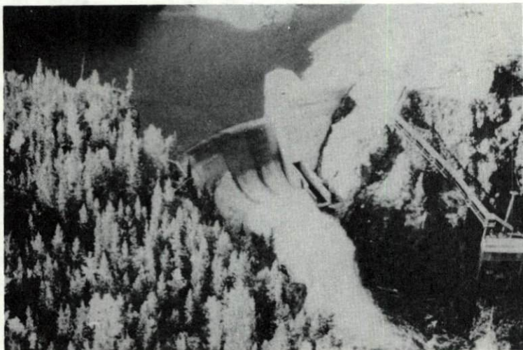
Impoundment dam at outlet of Fulton Lake.
