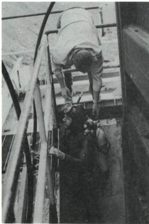
Diver preparing to inspect the Crofton Pulp Mill water intake screens: Cowichan River.
