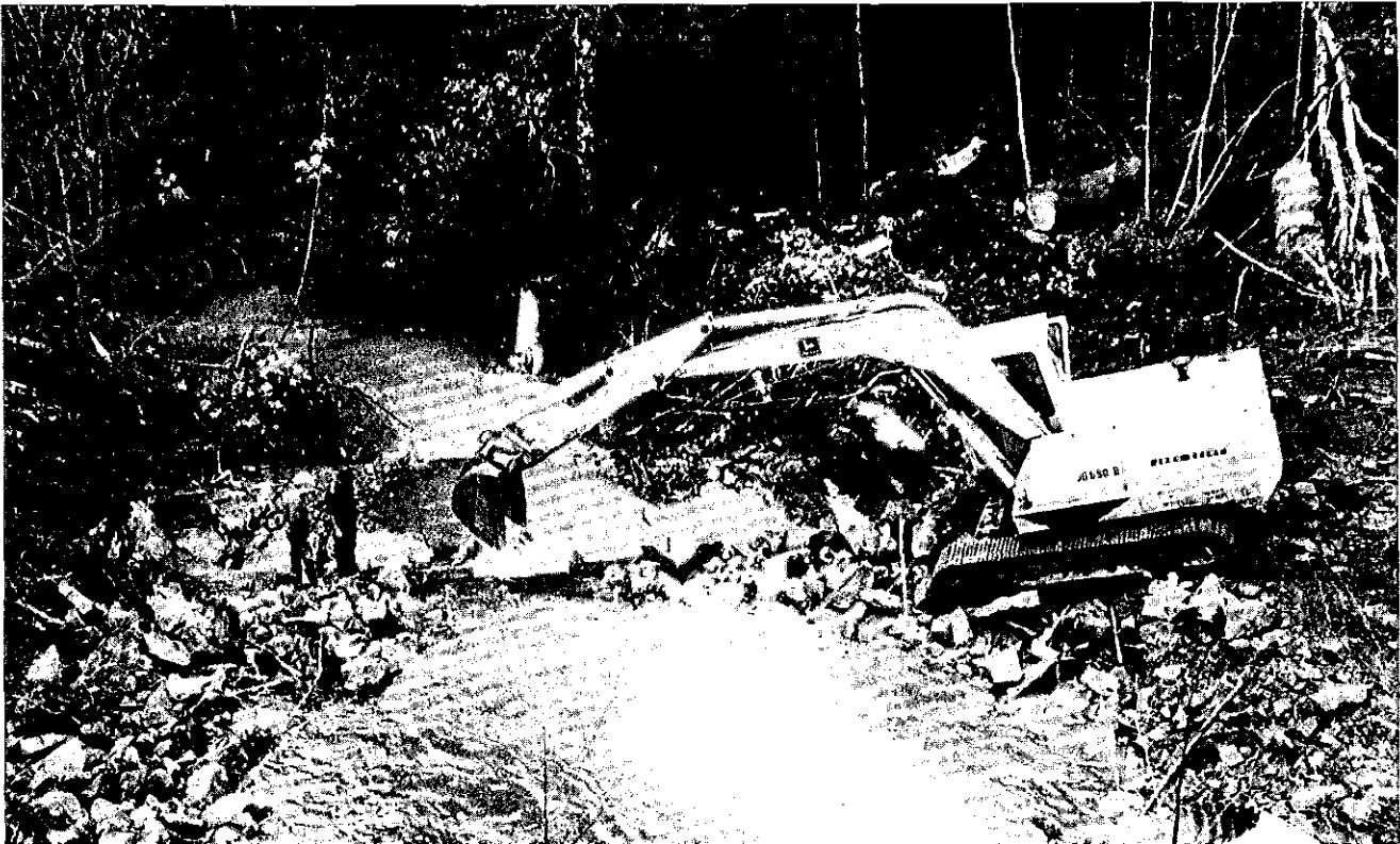
Building "steps" to facilitate fish passage to an improperly placed culvert on Chicago Creek, Hazelton.
