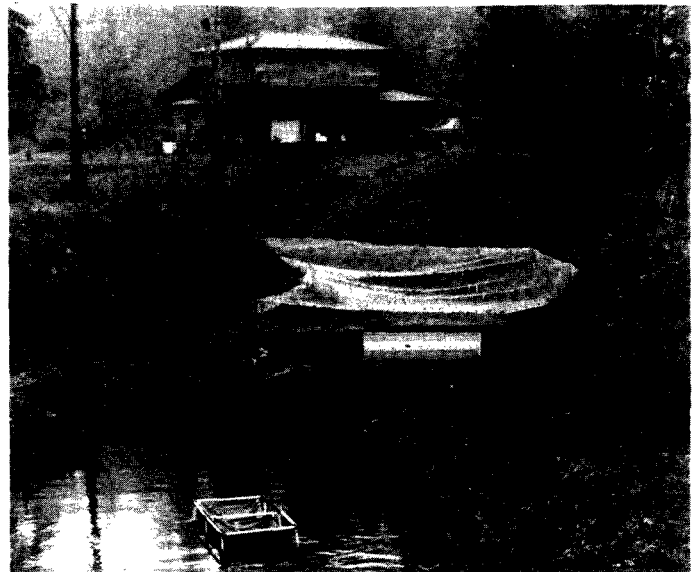
The main hatchery building overlooking the rearing channel was built at a cost of $6,000 and constructed of wood from the surrounding habitat.
