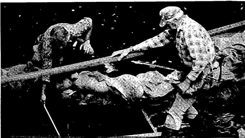
Two UIC workers make preparations for construction of a fishway on the Millstone River in Nanaimo.
