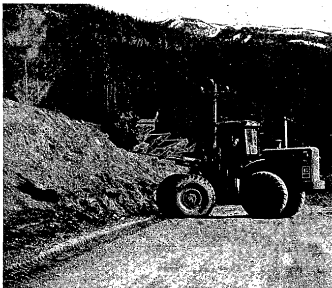
Loader prepares mine access road.
