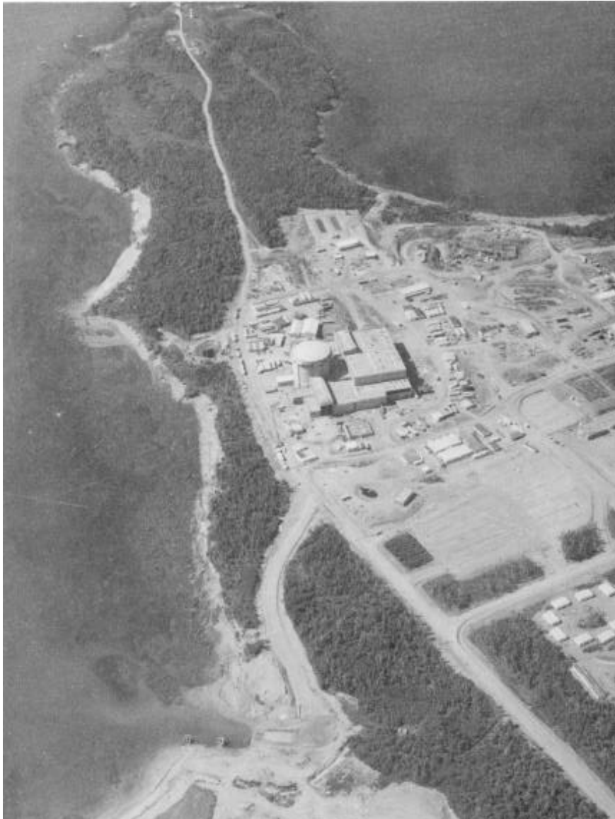
The Point Lepreau, NB, nuclear power generating station. Now over 60 per cent complete, the 630 megawatt CANDU station is scheduled to be in commercial operation at about the end of 1980. (Courtesy of the New Brunswick Electric Power Commission.)
