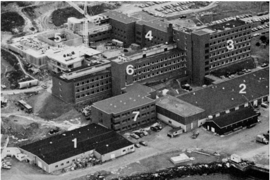
An aerial view looking east of the BIO complex. New facilities include: the Murray Building (4), which houses AGC and RMCB offices; the Holland Building (5), now under construction, that will house common services such as the library, computing Centre, and cafeteria; and the Strickland Building (7) where some MEL offices and laboratories are located. Older sections of the complex are the fish laboratory (1), Vulcan Building (2), Polaris Building (3), and Van Steenburgh Building (6). (BIO 5115-17)
