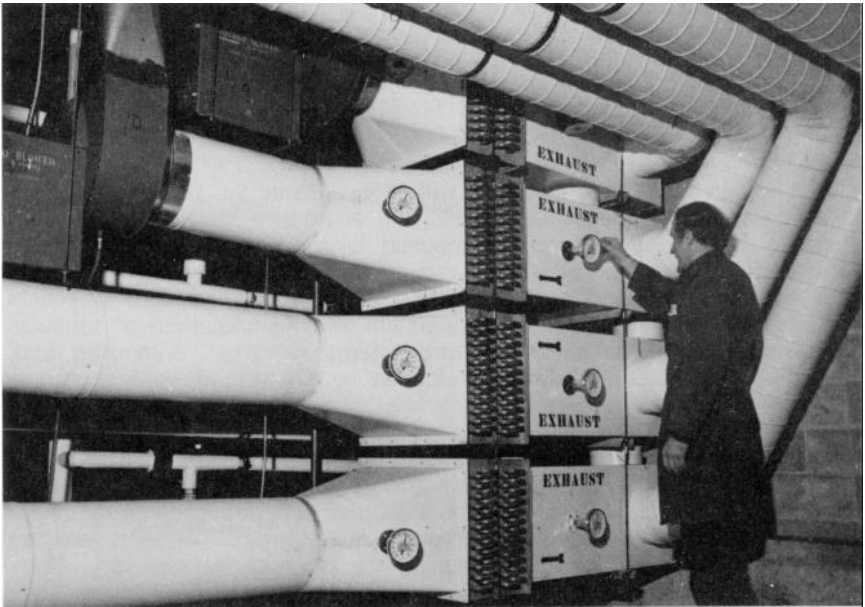
Buildings and Grounds staff of Engineering Services are responsible for routine building maintenance, heating plant maintenance, alterations, and additions. During the past two years senior staff of this group have acted as inspectors during the construction of the new buildings at BIO (see also Section F). Above, a tradesman checks that the heat recovery system is functioning properly. (BIO 5203-5)
