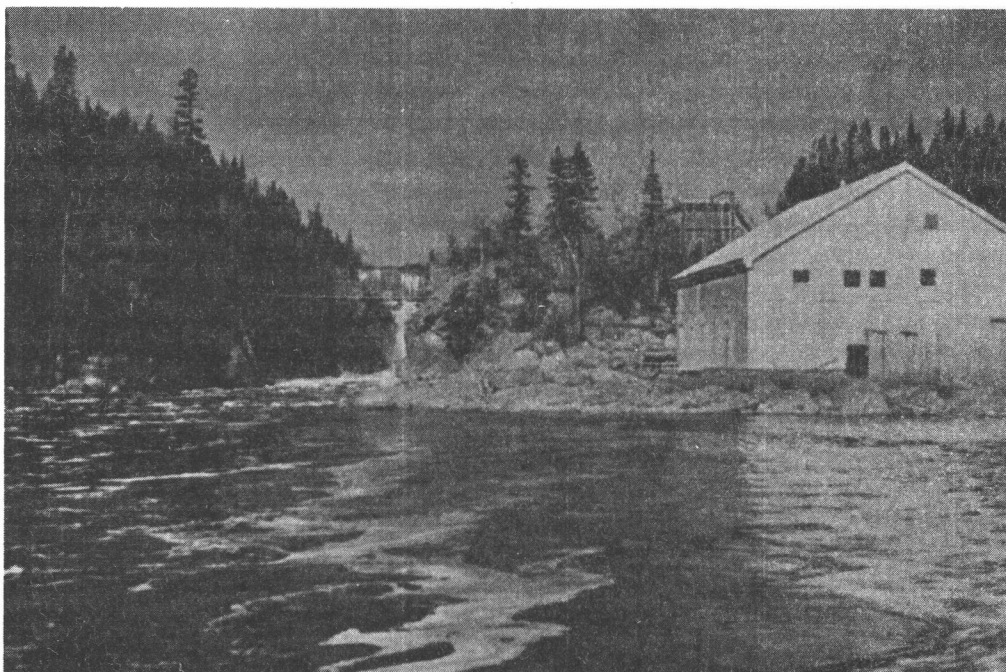
Liscomb hydro station, located downstream of the gorge below Liscomb Falls.
