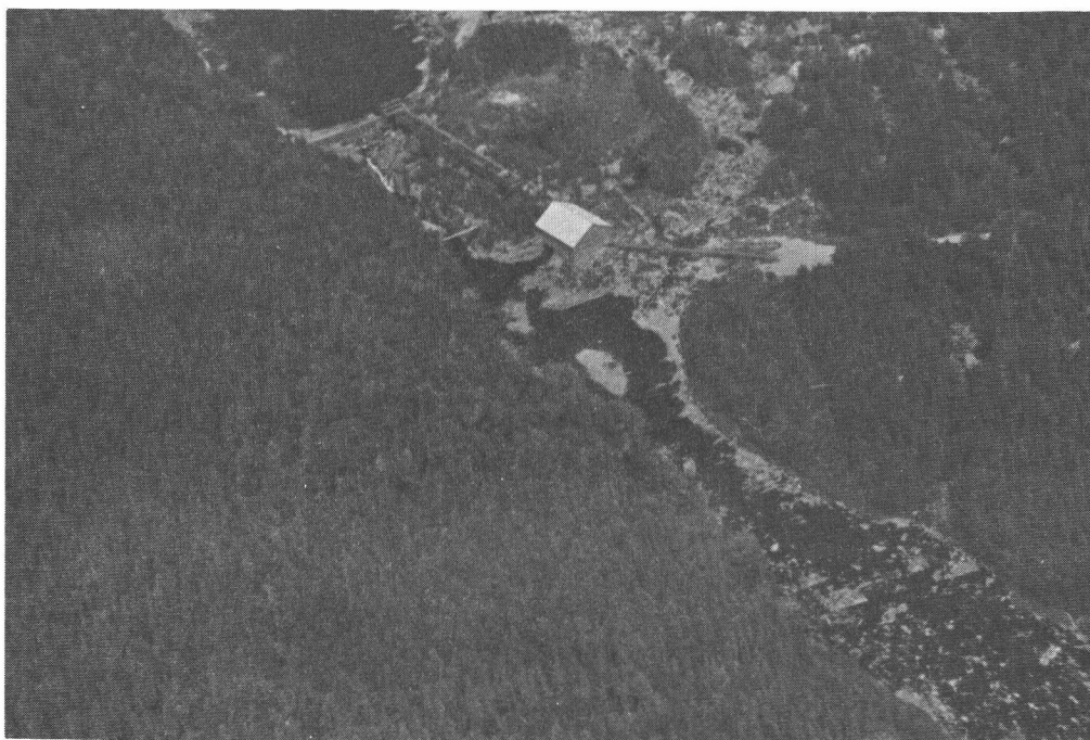
Aerial view of the Liscomb hydro site, showing headpond, main river dam, wing dam and hydro station.
