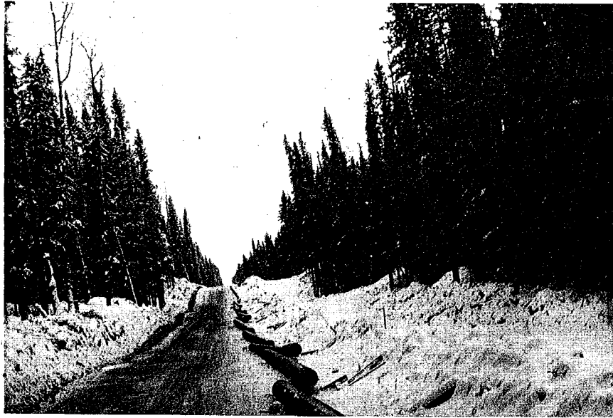
PLATE 4. The pipe "strung" along the right of way.
