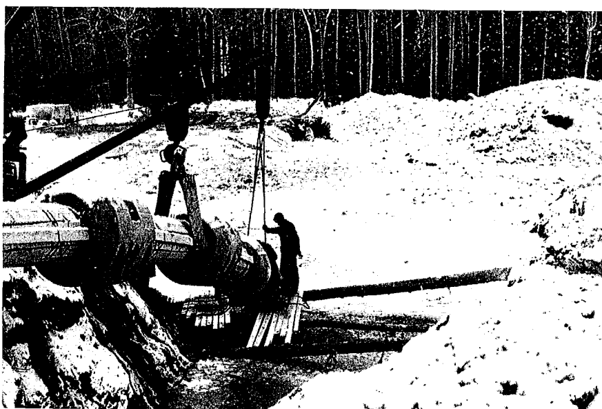
PLATE 20. Welding the strapped and weighted section of the pipeline to the existing pipe. Note the concrete collars to prevent floatation.
