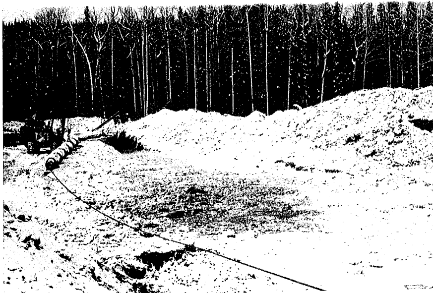
PLATE 18. Pulling the strapped and dressed pipe across the Kotaneelee River. Note the size of the crossing.
