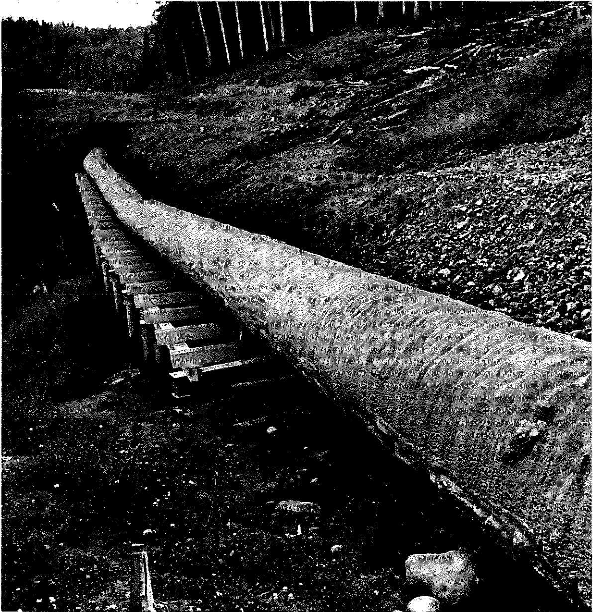
Figure 6: Exposed section of water supply pipeline to Fulton River Spawning Channel No. 2.
