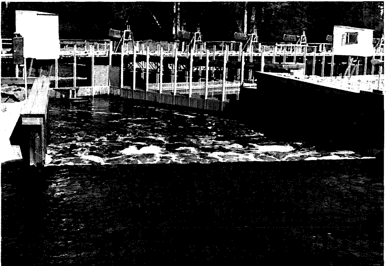
Figure 7: Adult and fry enumeration fence traversing the outlet of Channel No. 2 and Fulton River.
