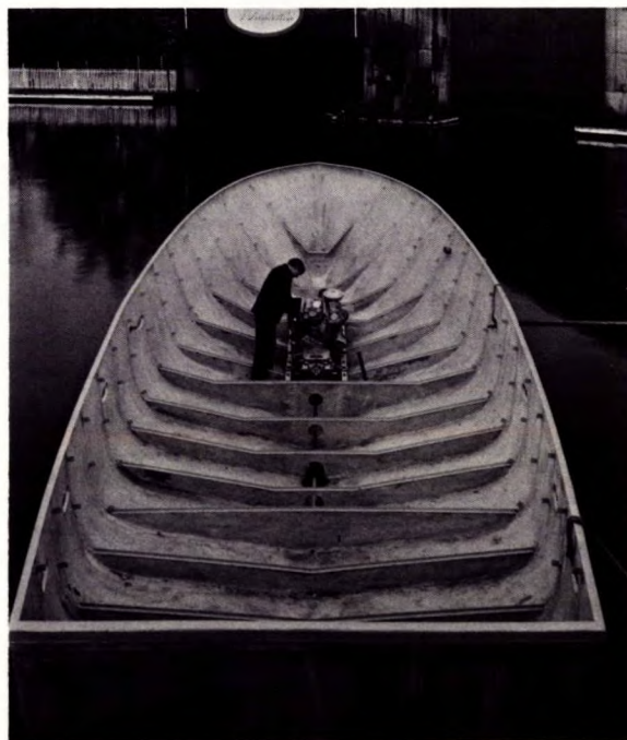
Photograph B. A 30-ft. Seacrete ferrocement hull with engine installed, as supplied to Kenya for completion locally into shrimp trawler. The hull maintains shape without cross bracing.
