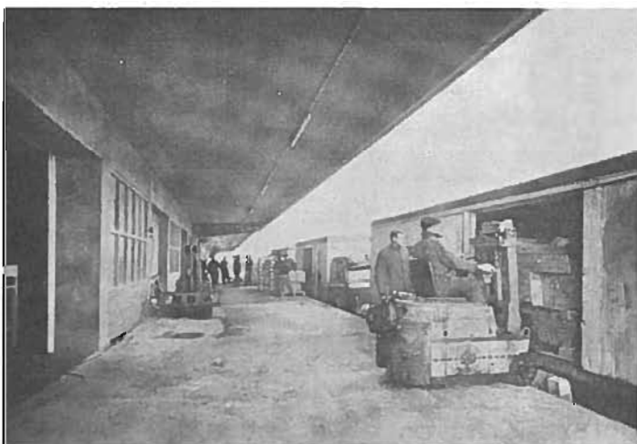
Cold Store Loading Dock for Trucks and Box Cars (Bremerhaven Cold Stores)
