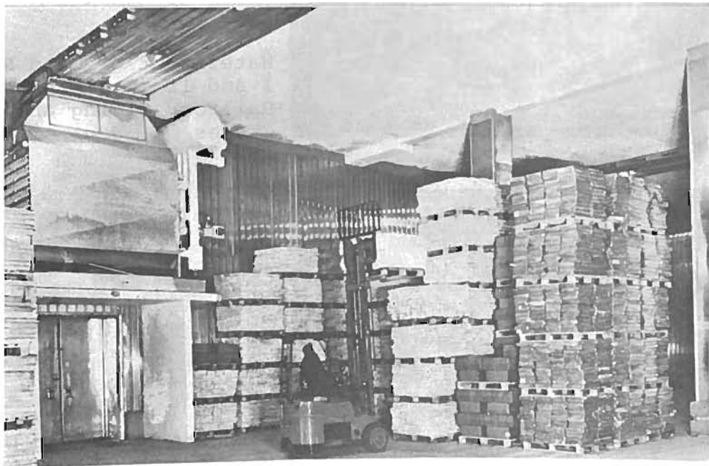
Interior of One of the Cold Storages, Max. Stacking Height Approx. 23 Feet (Bremerhaven Cold Stores)
