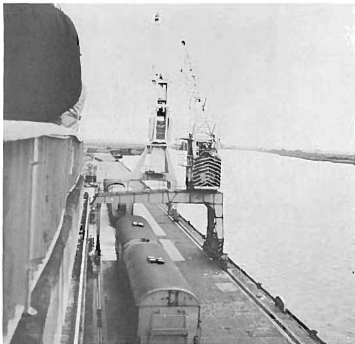
Cold Stores' Waterfront with Siding and Unloading Cranes
