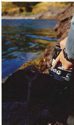
Installing a Shore Fastening
