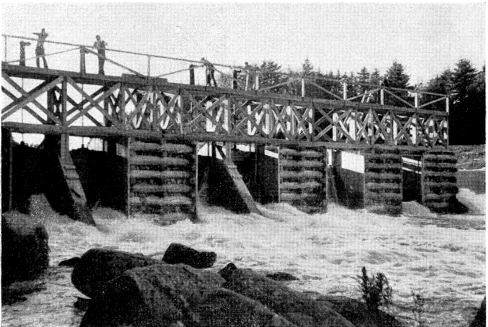
FIGURE 7. Wentzell's Lake dam seen from below during production of a freshet. Four men on top of the dam are raising the freshet gates by hoists. The fifth opening from the left is a log-driving gate, not used in the experiments. The opening at extreme right is a fishway and beyond it the spillway.
