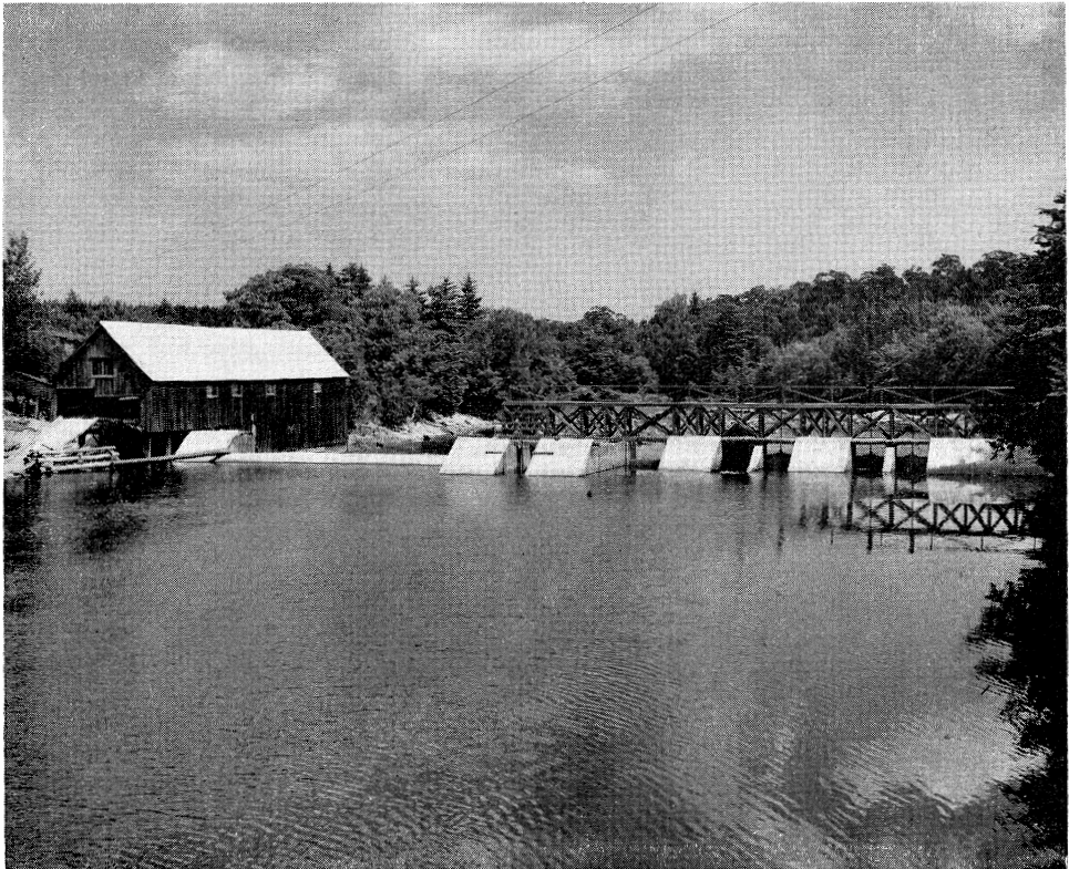
FIGURE 4. Freshet-production dam at Wentzell's Lake, seen from above. To the left is the mill which uses the stored water for power at certain times of year. The wide opening to the right of the mill is the spillway, and then a fishway, log driving gate and two double freshet gates. To produce a freshet the gates are raised by four hoists on top of the dam.
