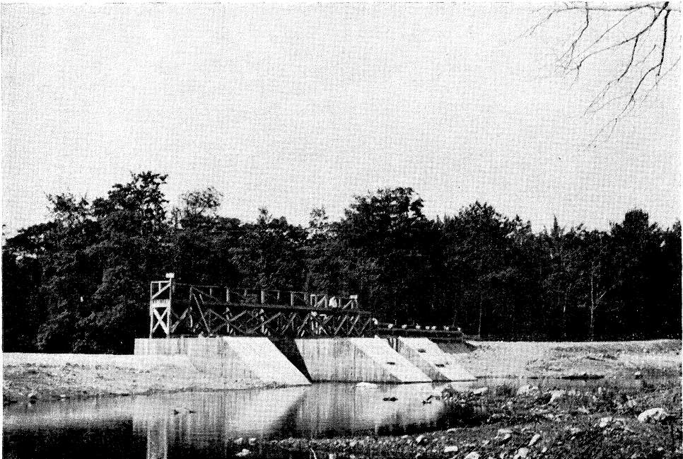
FIGURE 3. Sherbrooke Lake storage dam seen from above. There is a double gate at centre, raised and lowered by two gate hoists. The dam also contains a fishway, and there is a lumber-driving gate. A head of six feet of water over an area of seven square miles is maintained by the dam.
