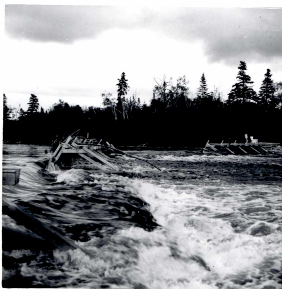
Fig. 13. Fence washout at Harry's River.
