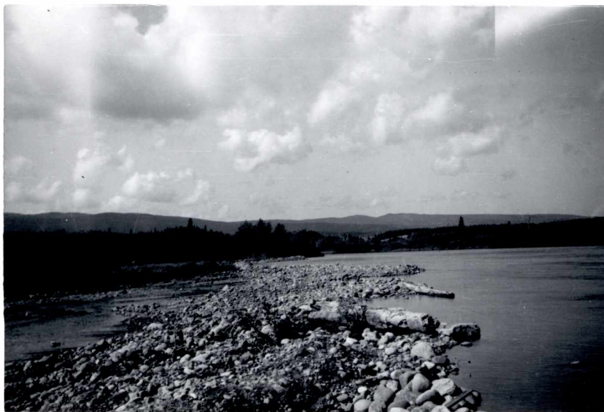
Fig. 12. Rock dyke at Harry's River.
