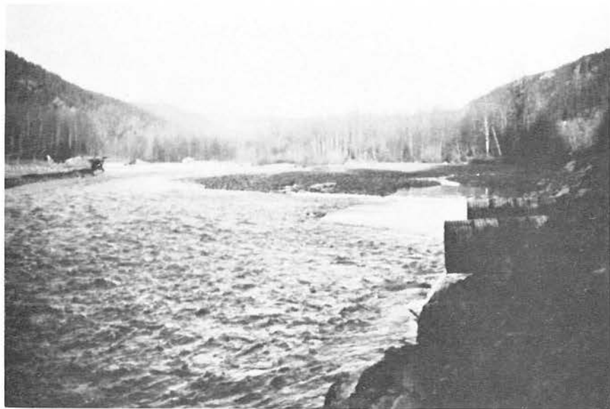
Figure 10. Log jam at outlet of Mosley Lake (upper) and culvert through which Tenderfoot Creek enters the Cheakamus River (lower).
