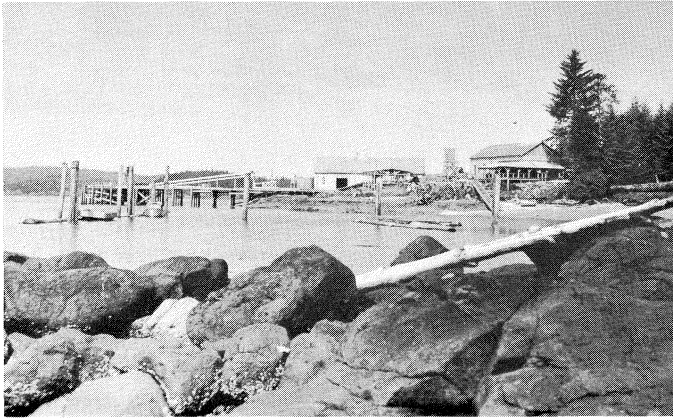
FIGURE 30. Wharf and processing plant of Canada Kelp Company Limited, on Deer Island, near Hardy Bay, British Columbia, in 1947.
