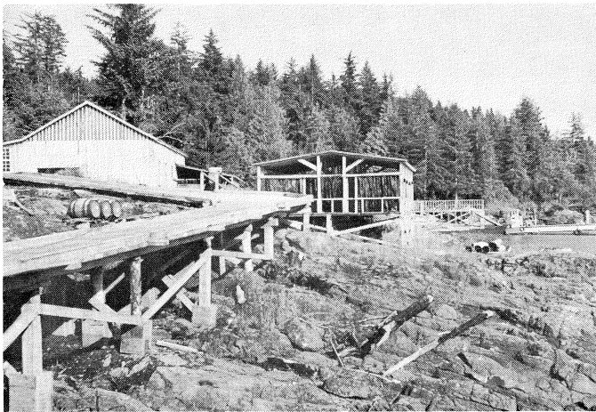
FIGURE 31. Powerhouse and pilot plant of the same plant as Fig. 30, showing outdoor drying racks and (right background) the converted landing-barge used as a harvester.
