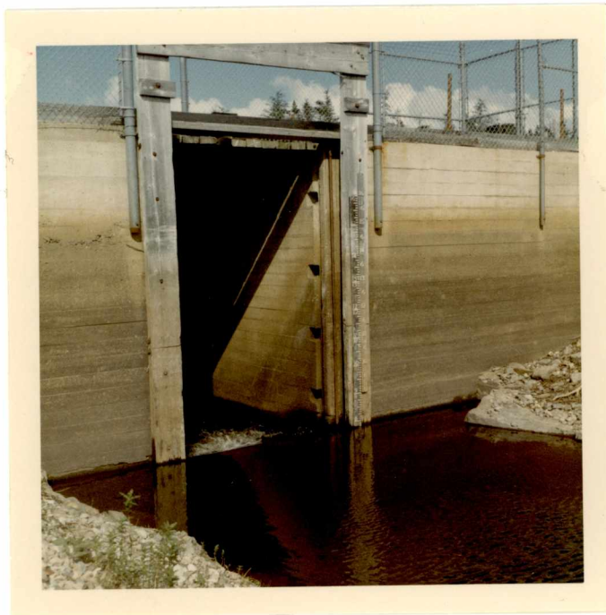
Fig. 4. Controlled flow spillgate at the outlet of Thomas Pond.
