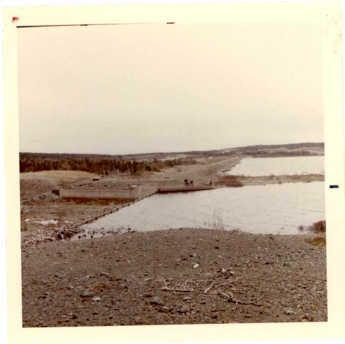
Fig. 3. Thomas Pond dam and high-water spillway.
