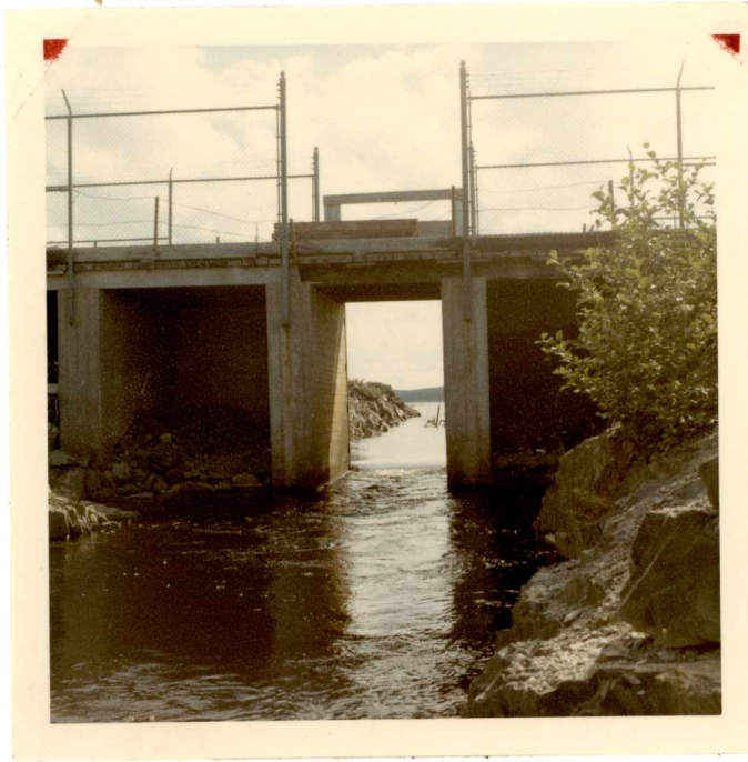
Fig. 5. Diversion channel leading into the Topsail River system.
