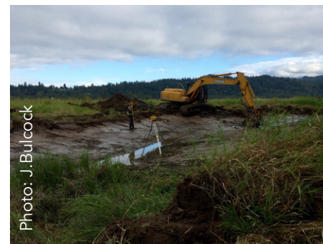
FVWC and DFO begin tidal channel restoration. Low shallow-grade benches are being created to support native aquatic sedge and plant communities.
