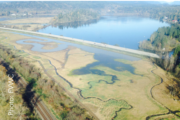
Stave River (2016) looking west along the lower Stave River off-channel habitat project site. At this site, new ground-water fed channels were created, fish barriers were removed and efforts to mimic the natural draw-down of water were established.
