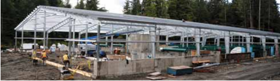
'Namgis land-based recirculating aquaculture system under construction. Photo: Jackie Hildering (K'udas Limited Partnership)
