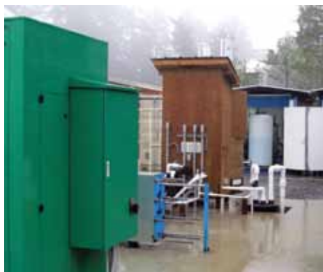
Marine Hatchery Water Conditioning Module (water chiller, monitoring and control panel, alarms, reverse osmosis equipment). Photo: Linda Hiemstra (Sable Fish Canada Ltd.)
