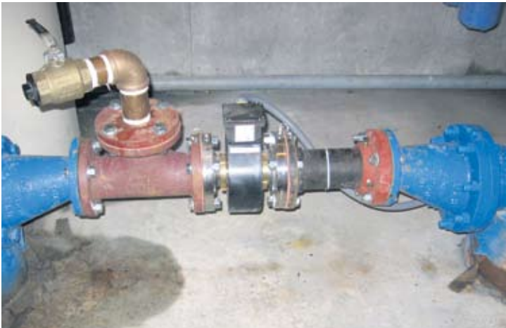
MagFlow Water Meter Assembly (Photo: D. Bevan)
